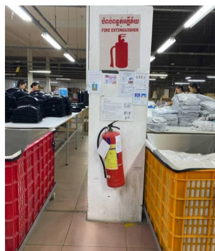
Photo: 7 Nov, 2023 – A fire extinguisher is mounted on a column in a garment factory with a clear sign to enhance visibility and accessibility in case of a fire emergency.
