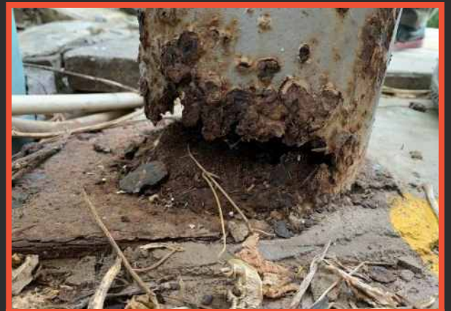
Corroded steel column
