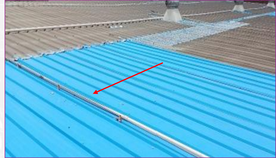
Eearthing provided to MS truss
