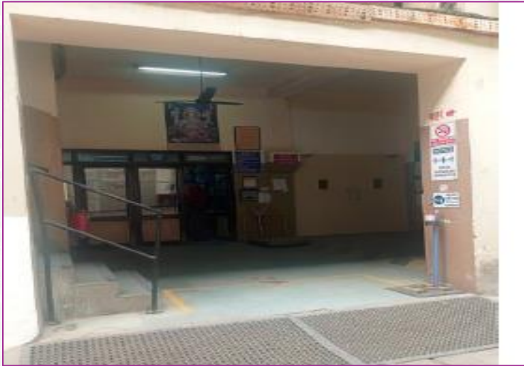
Rolling shutter has been removed
