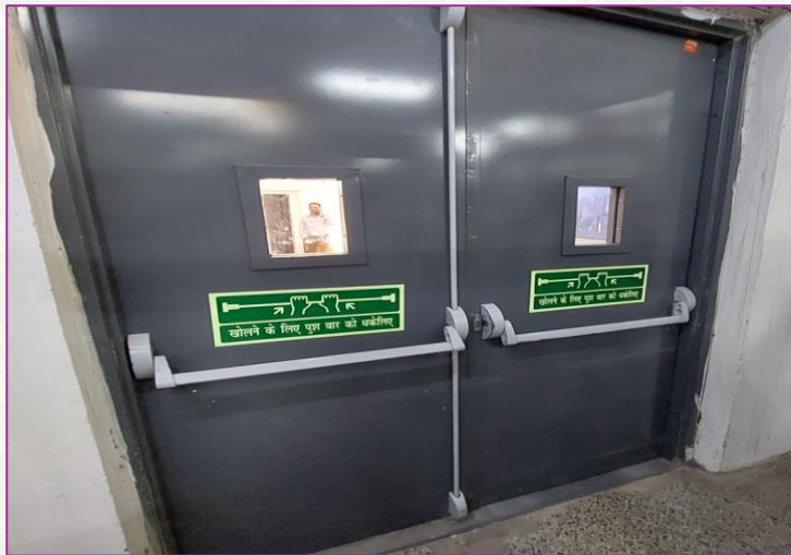
Push bar has been install over doors
