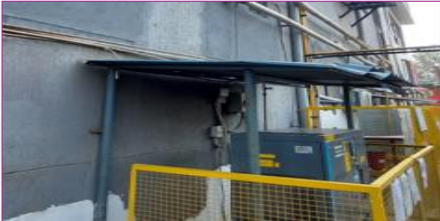
Window opening towards compressors has been closed
