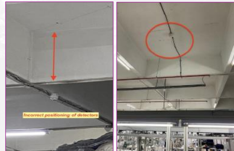
Smoke detector positioning before and after
