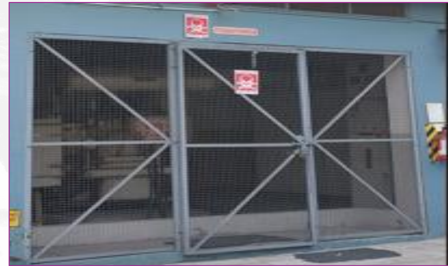
Warning signage provided
