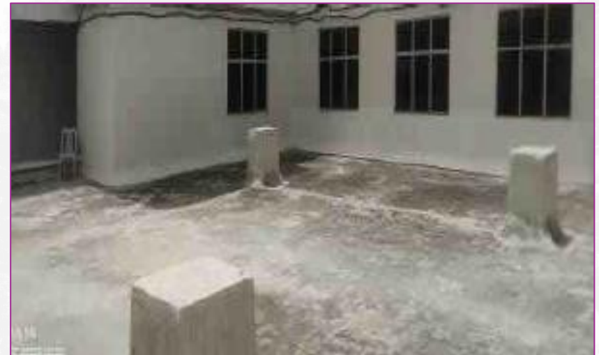
Corroded bars were repaired from column
