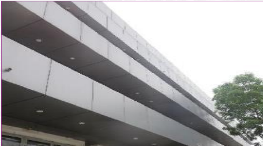
Corroded structure repaired and covered
