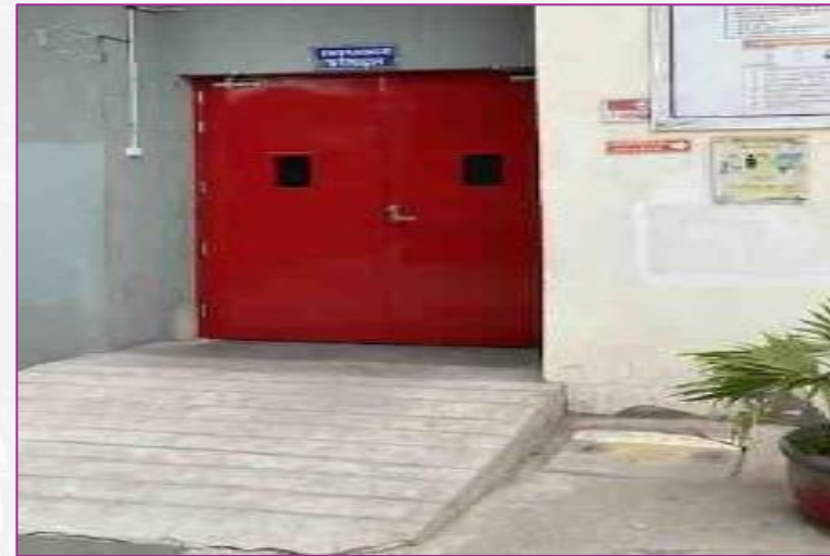
Fire door has been installed
