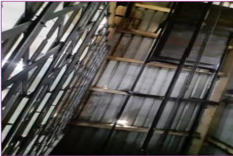
Structural member has been reinforced
