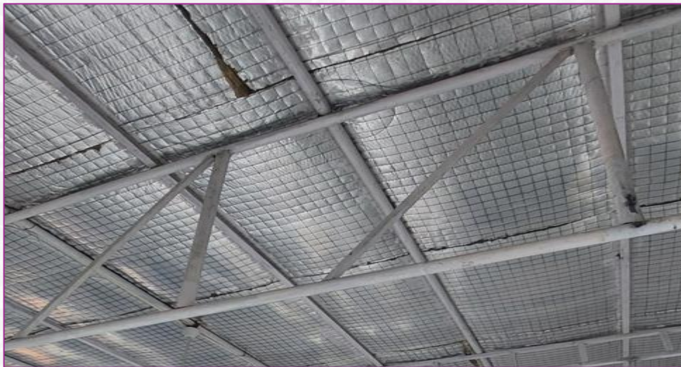
Bracing to MS structure
