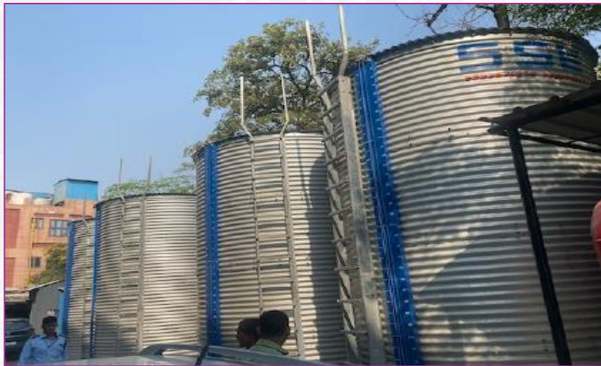
Additional water tanks installed by factory
