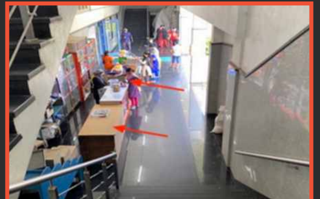
Exit passage blocked by vending counter
