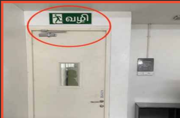
illuminated exit sign not provided over exit
