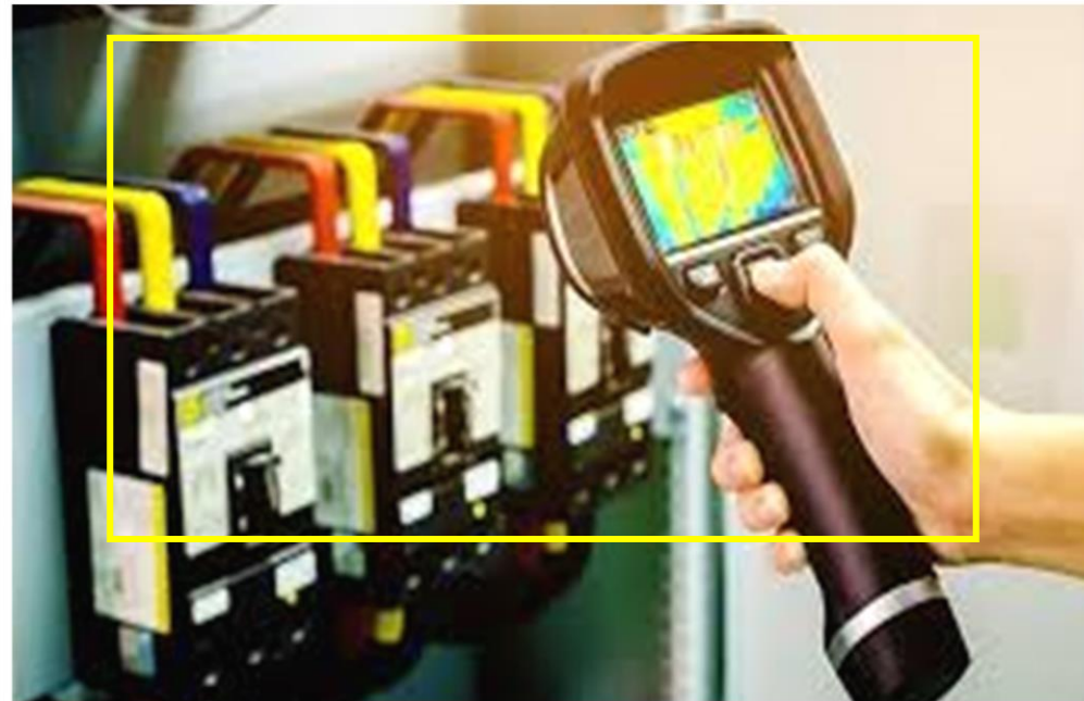
Monitoring of electrical panel temperature
