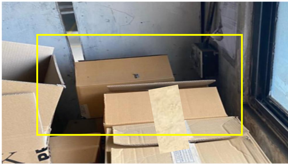
Material stored incorrectly and near Electrical source
