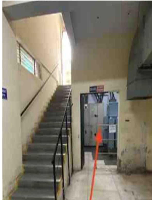
Hazardous installation in escape route
