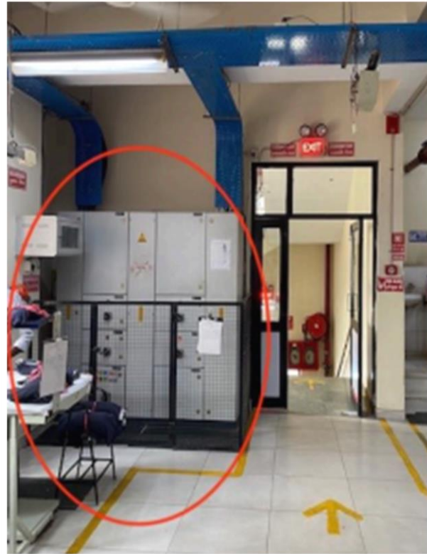
Electrical fixture in escape route
