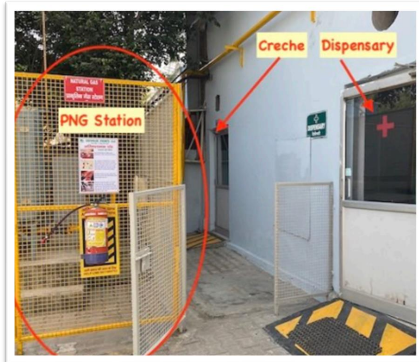
High risk installation without segregation
