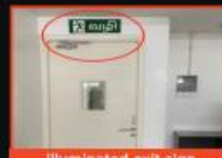
Illuminated exit sign not provided over exit
