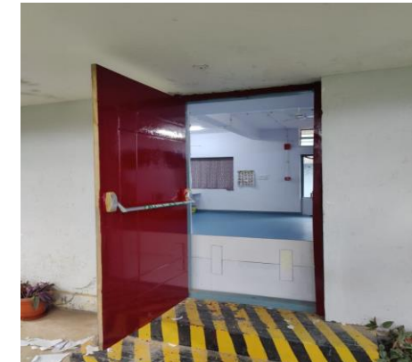
Door with panic bar provided at emergency exit
