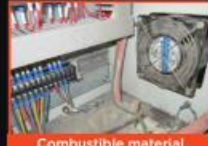
Combustible material inside electrical panel
