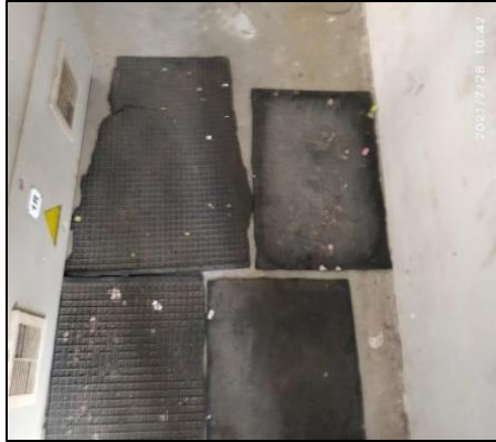
Insulated rubber mat were worn out
