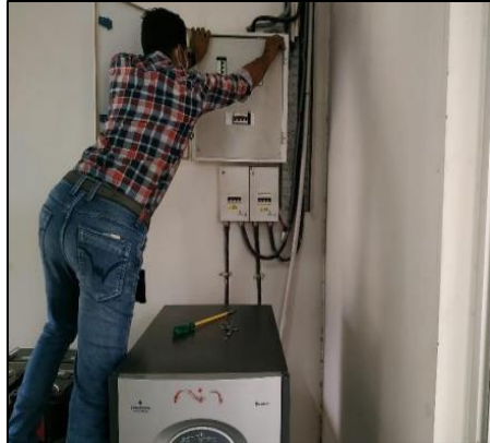
The distribution board were not accessible
