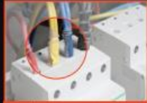
Lint/dirt on electrical panel
