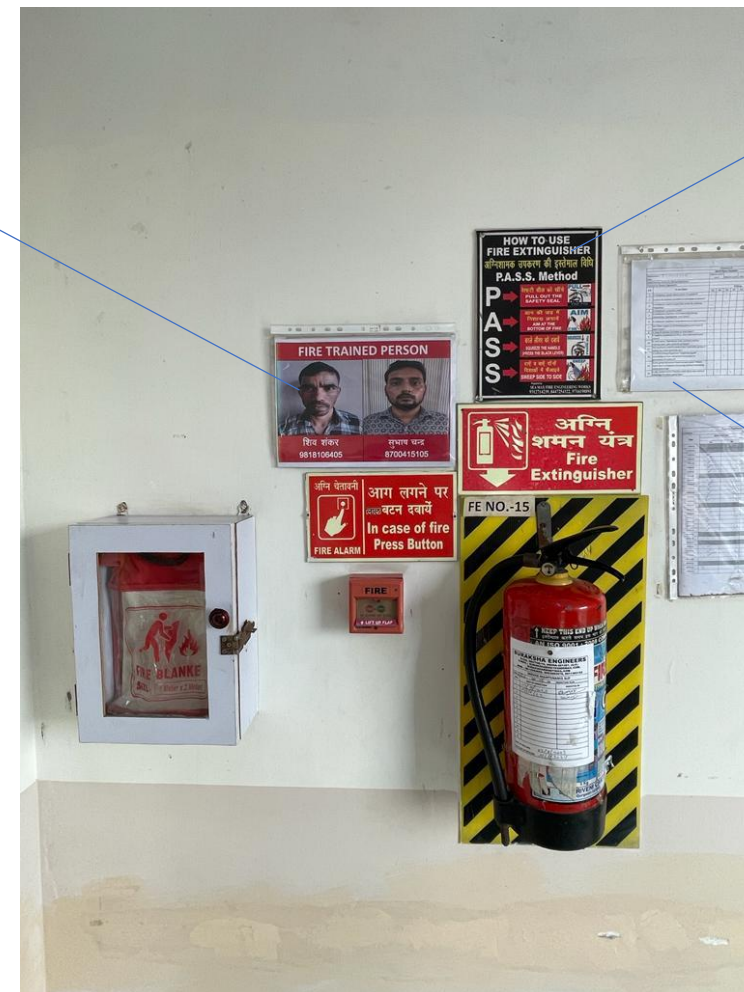
Fire Extinguisher, MCP & Blanket
