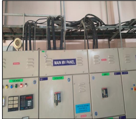
Electrical wiring and cables not properly identified
