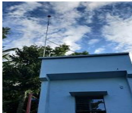
LPS Installed at factory after risk assessment
