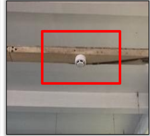
Smoke detectors and heat detectors not installed on the ceiling or roof
