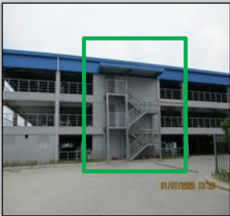
Exterior exit stairs separated from building interior by 3.1 m beyond the ends of the stair structure
