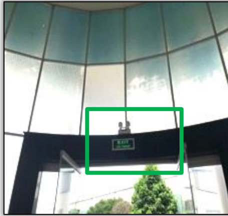
illuminated exit signs provided above each emergency exit door
