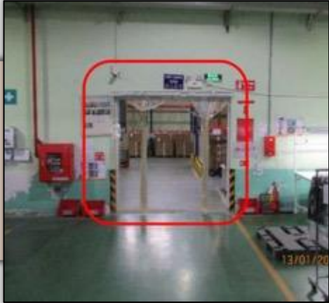
Fire rated doors not installed
