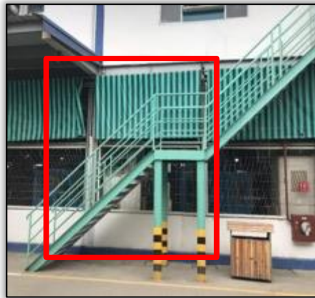
Exterior exit stairs not clear of building interior by 3.1 meter
