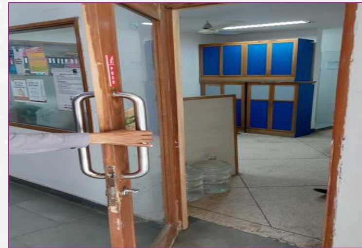
Rotating latch mechanism installed to bypass lock
