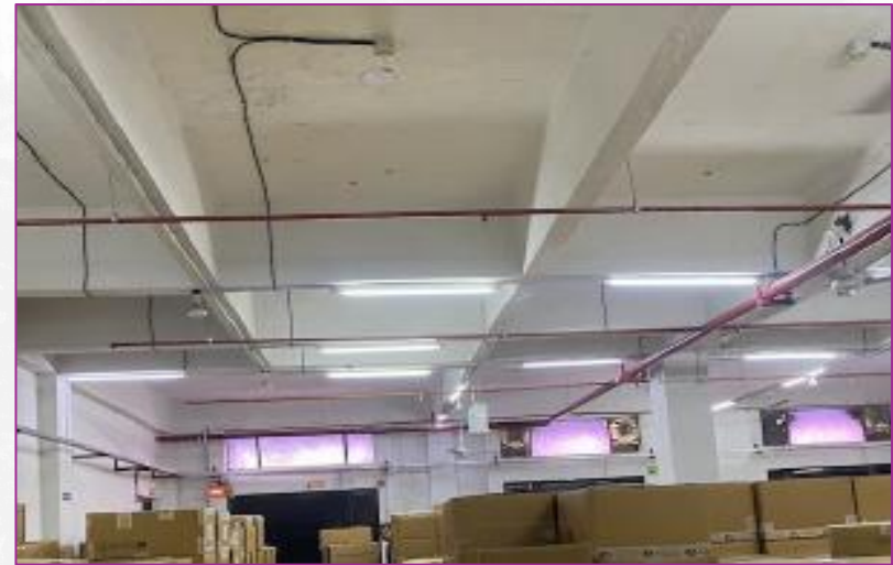
Sprinklers installed in material store
