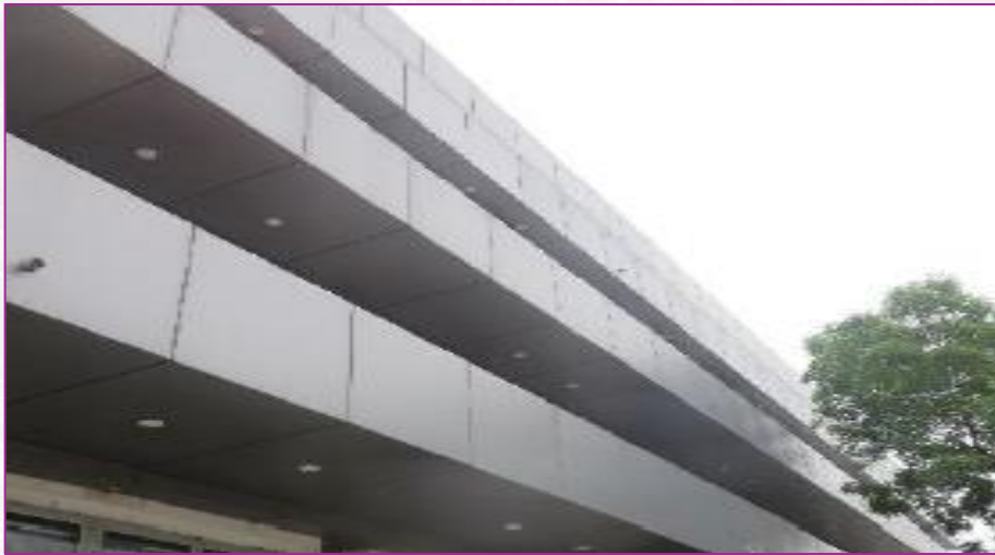
Corroded structure repaired and covered
