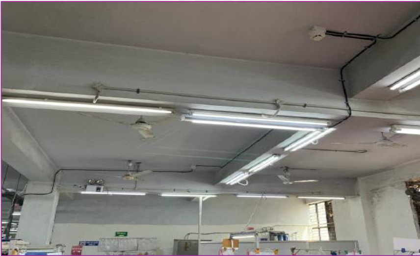
Smoke detector installed
