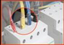
Lint/dirt on electrical panel
