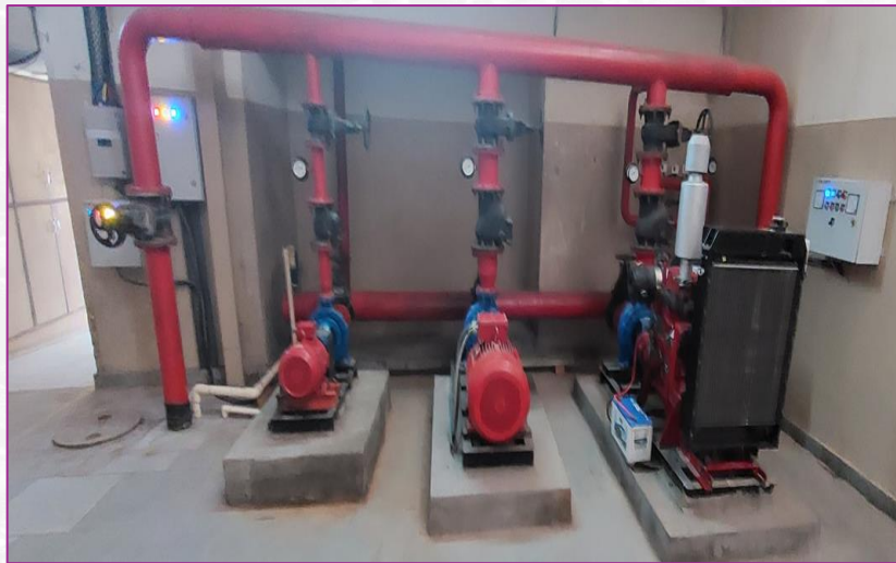
All 3 Fire pumps are installed
