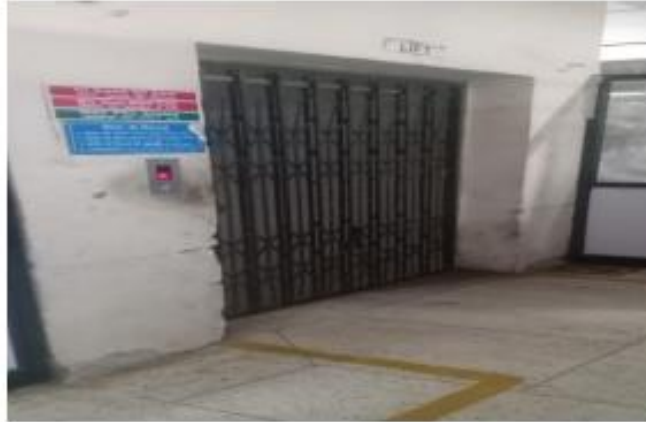
No separation of lift shaft
