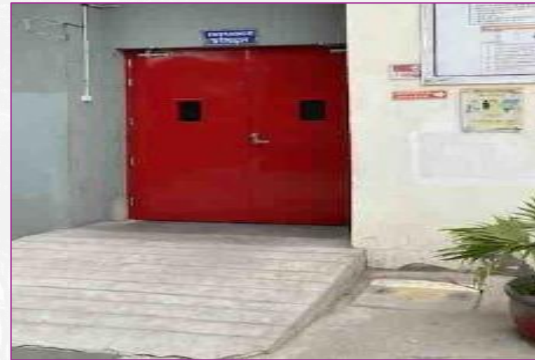
Fire door has been installed
