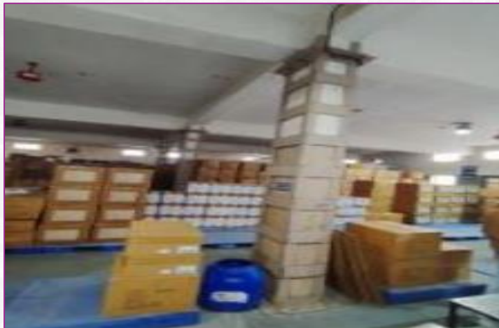
Jacketing provided for column level below
