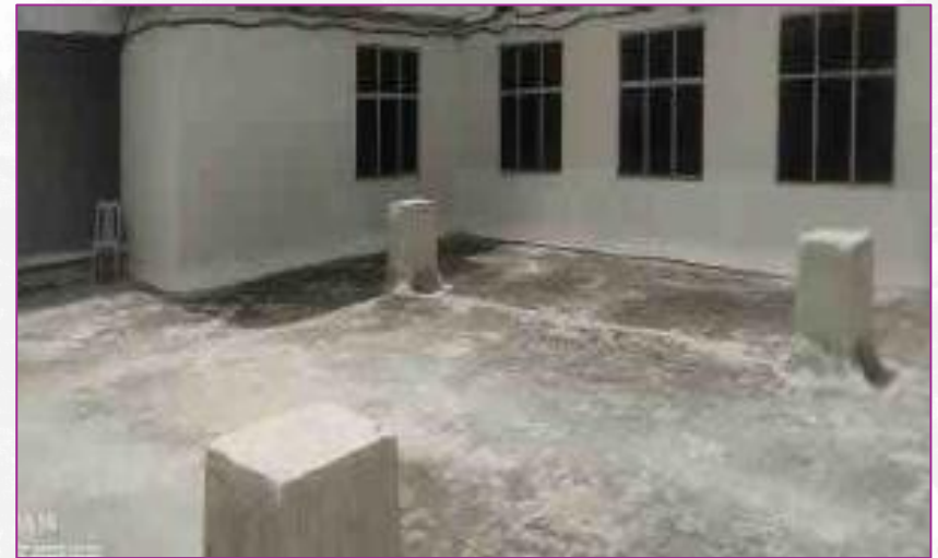
Corroded bars were repaired from column
