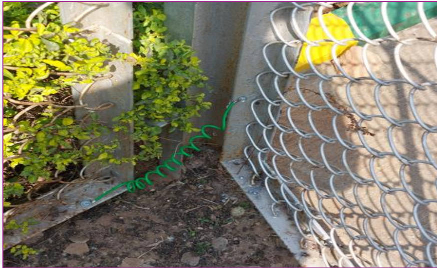
Bonding provided over transformer gate
