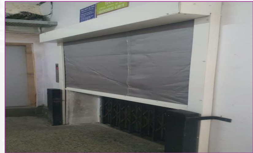
Panel room enclosure by fire door
