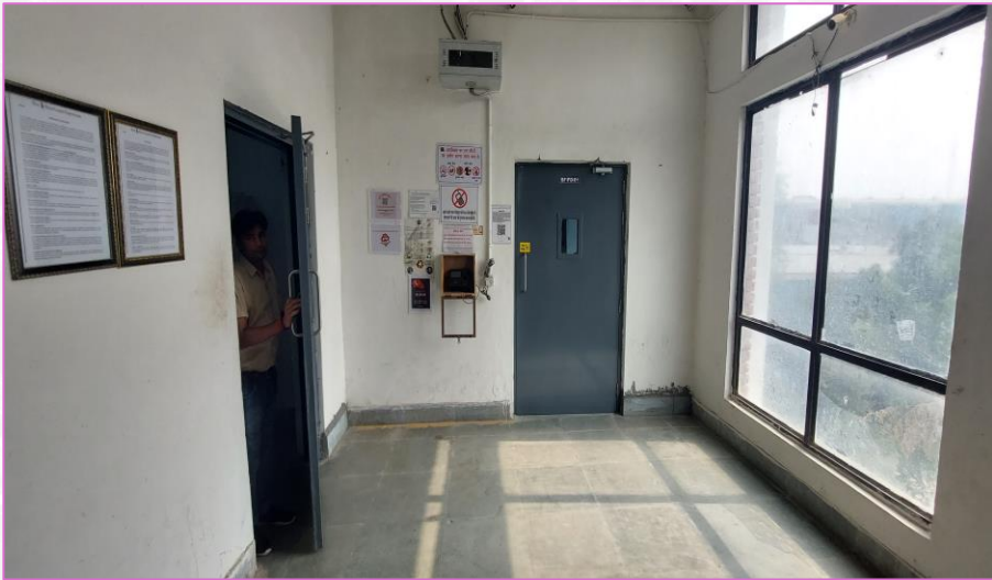
Staircase compartmentation with Fire doors
