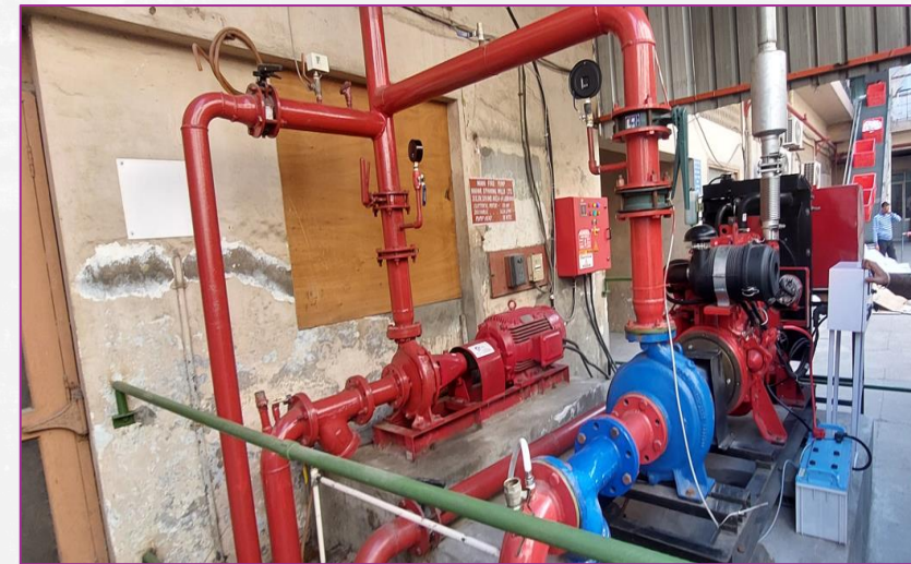
Backup Fire pumps are installed
