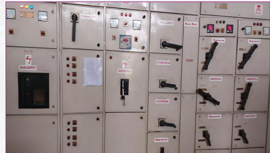
Proper identification provided over panel
