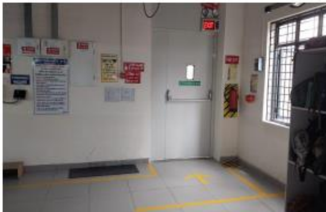
Fire rated door with push bar
