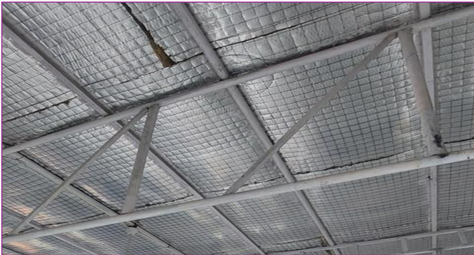
Bracing to MS structure
