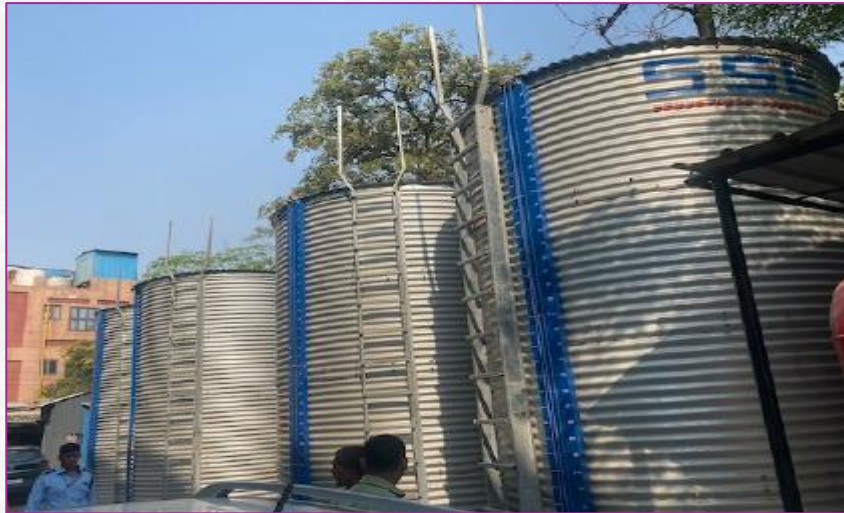
Additional water tanks installed by factory
