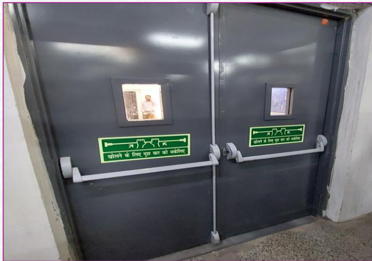
Push bar has been install over doors
