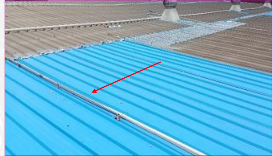
Eearthing provided to MS truss
