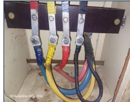
Replaced Rusted Nuts and Bolts in Electrical Installation
