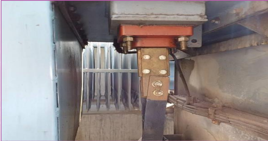
double Earthing provided to transformer
