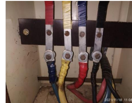
Rusted Nuts and Bolts In Electrical Installation
