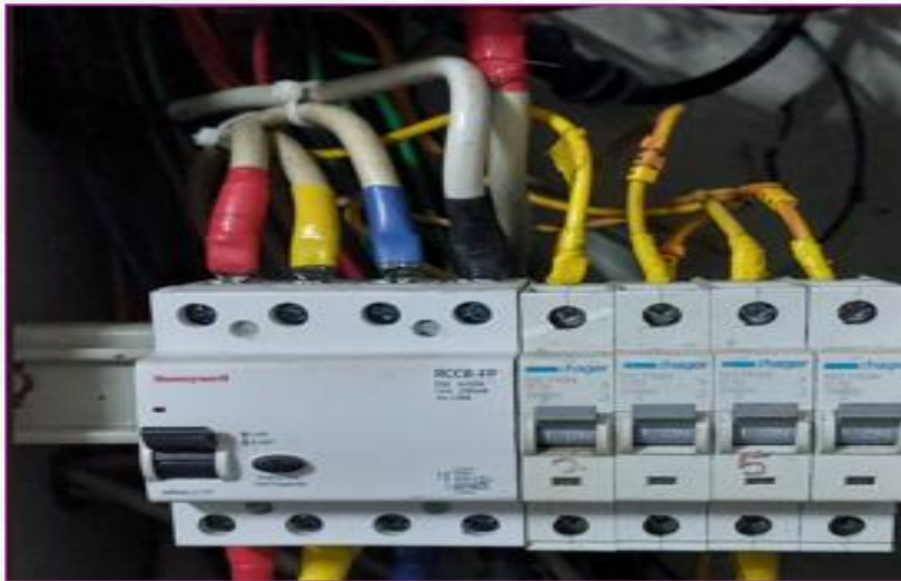
Lugs provided for electrical panel
