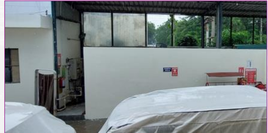
Wall separation provided between transformer & evacuation route
