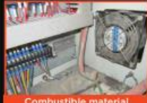
Combustible material inside electrical panel
