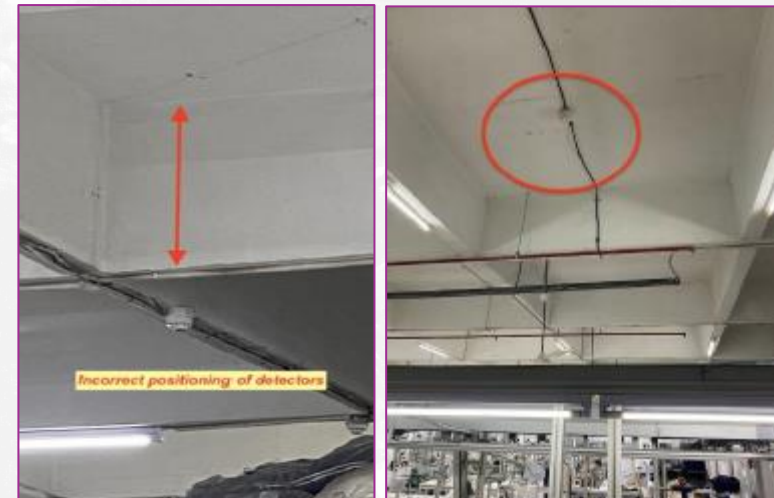
Smoke detector positioning before and after
