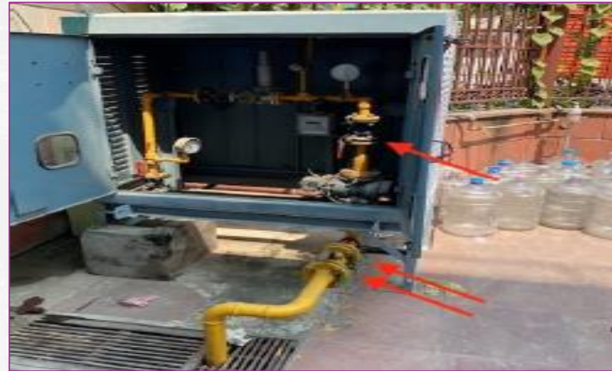
Bonding provided over LPG gas pipeline
