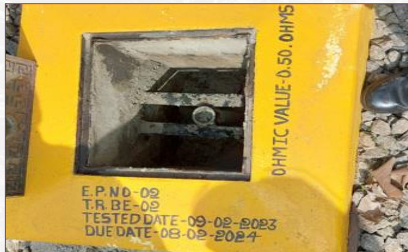
Earth pit maintained and monitored
