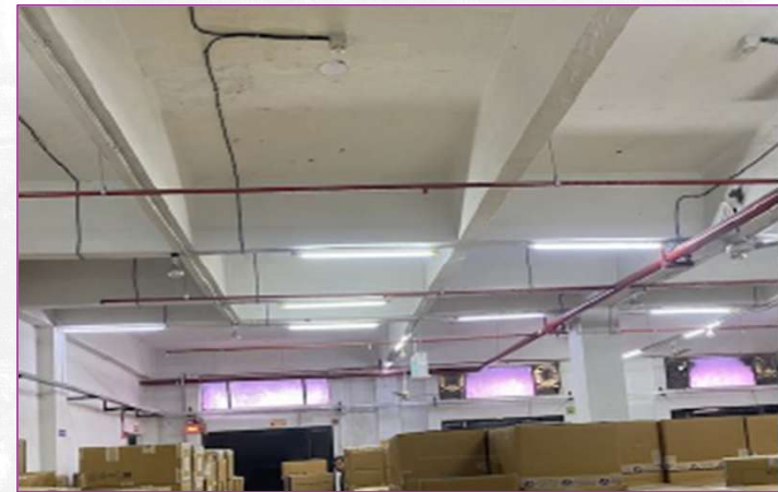
Sprinklers installed in material store
