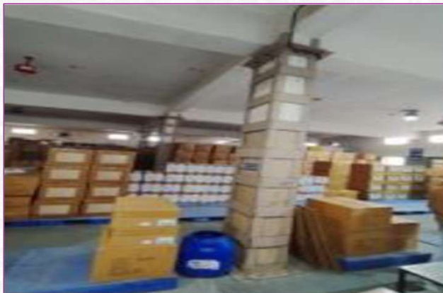
Jacketing provided for column level below
