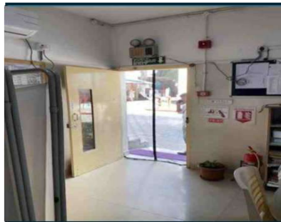
Illuminated Exit Signage Insatlled
