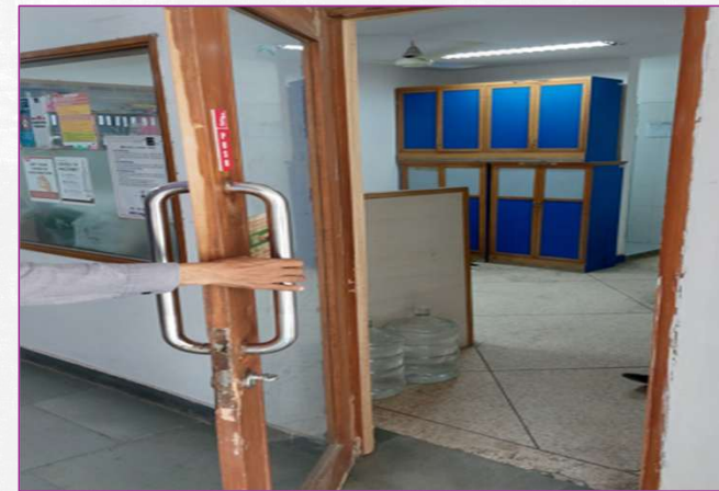
Rotating latch mechanism installed to bypass lock
