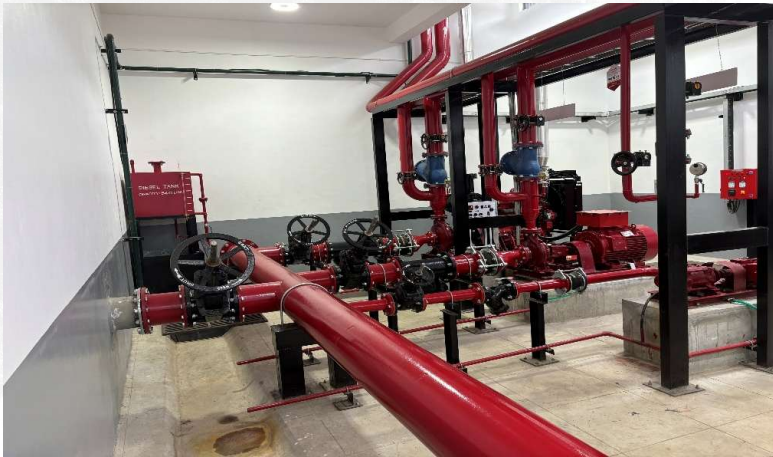
All 3 Fire pumps are installed
