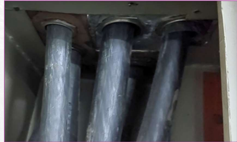
Glands provided over electrical panel
