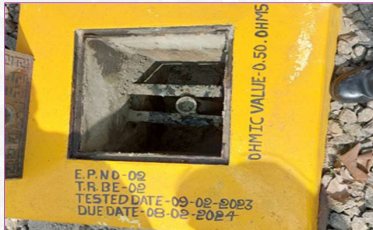
Earth pit maintained and monitored.
