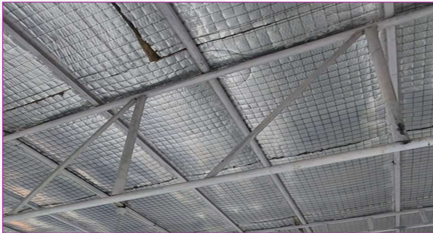
Bracing to MS structure
