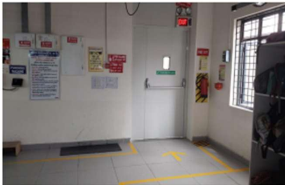
Fire rated door with push bar
