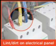
Lint/dirt on electrical panel
