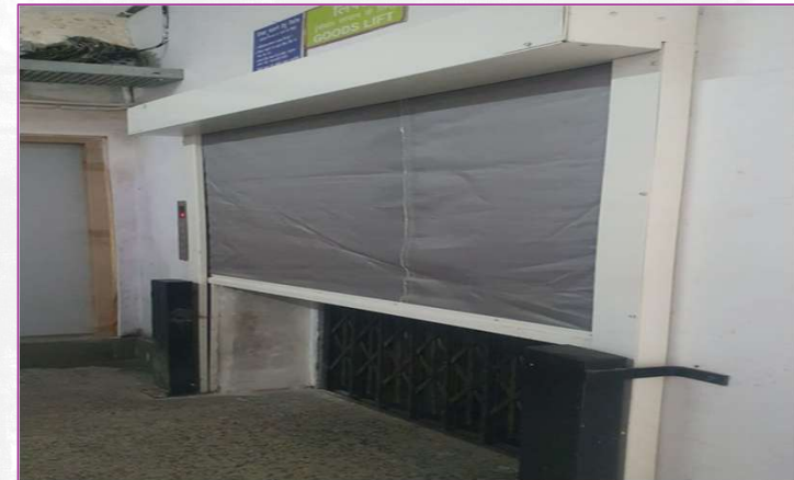
Panel room enclosure by fire door
