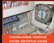
Lint/dirt on electrical panel
