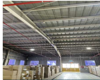
Storage Area With Sprinkler System
