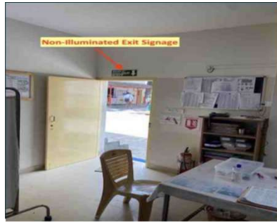
Non Illuminated Exit Signage Insatlled
