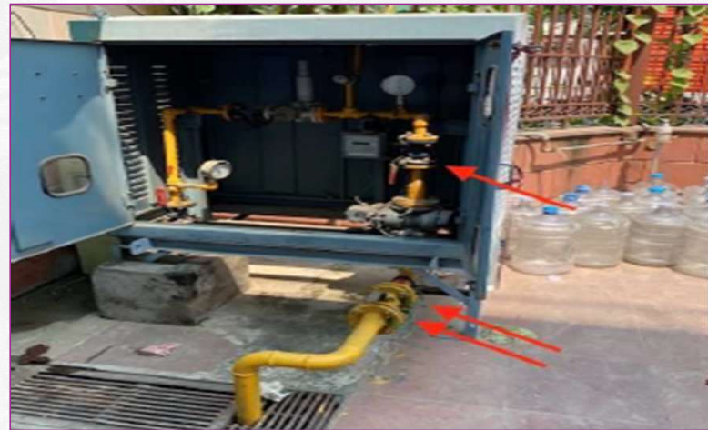
Bonding provided over LPG gas pipeline
