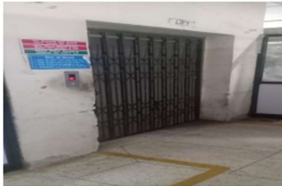
No separation of lift shaft
