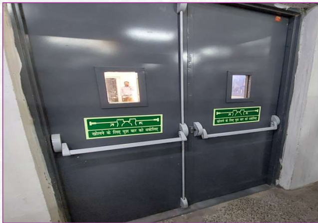
Push bar has been install over doors
