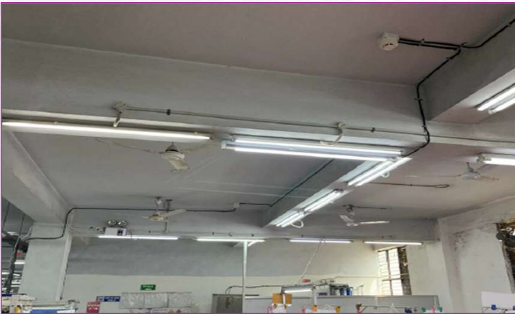
Smoke detector installed
