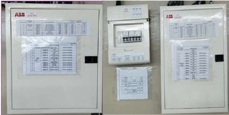
Current carrying capacity calculated and posted over DB
