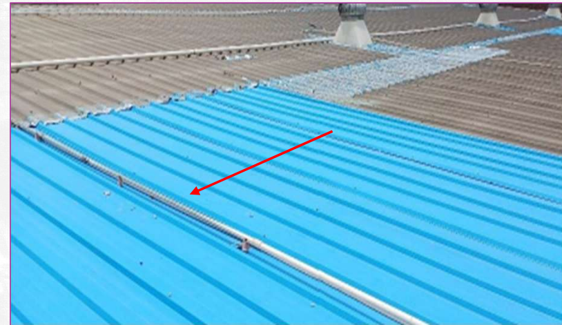
Eearthing provided to MS truss
