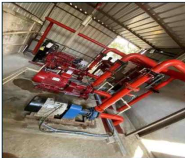
Hydrant Pumps installed
