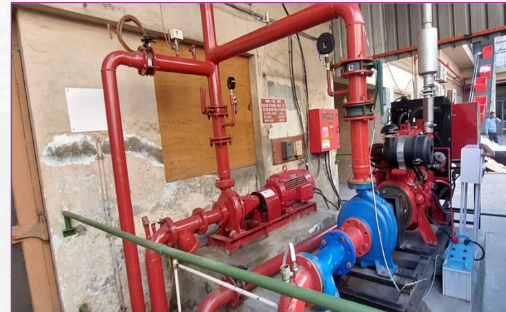
Backup Fire pumps are installed
