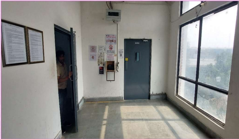
Staircase compartmentation with Fire doors
