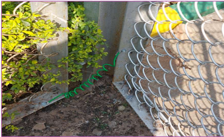
Bonding provided over transformer gate
