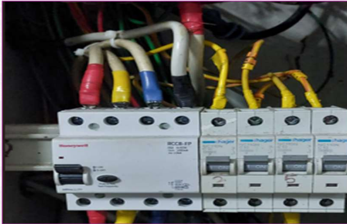
Lugs provided for electrical panel
