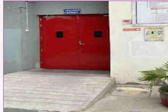
Fire door has been installed
