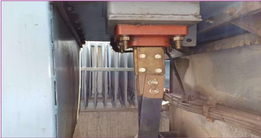
double Earthing provided to transformer
