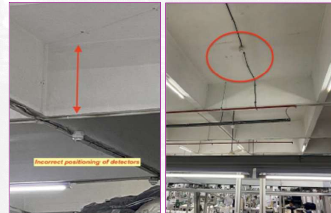
Smoke detector positioning before and after
