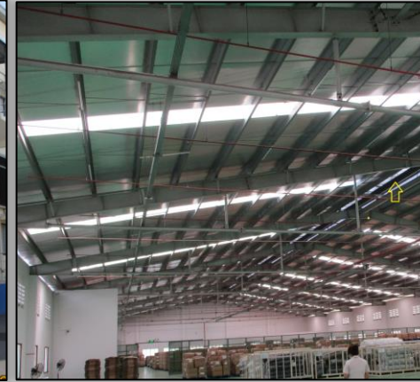
The sprinkler heads were far away ceiling
