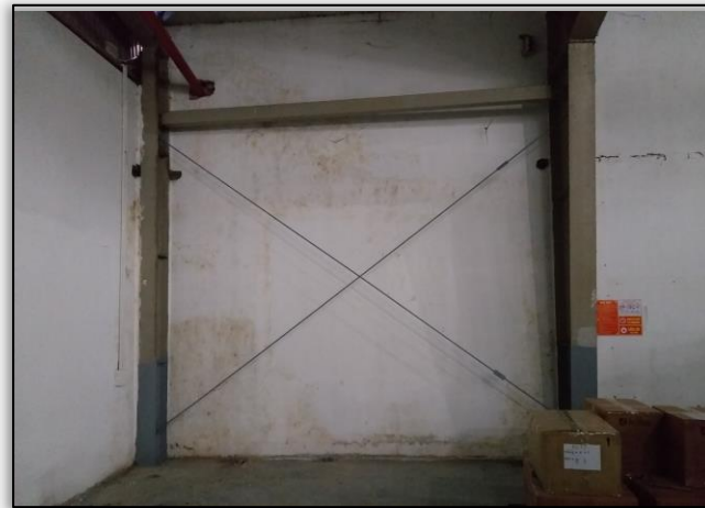
The column bracings have been installed
