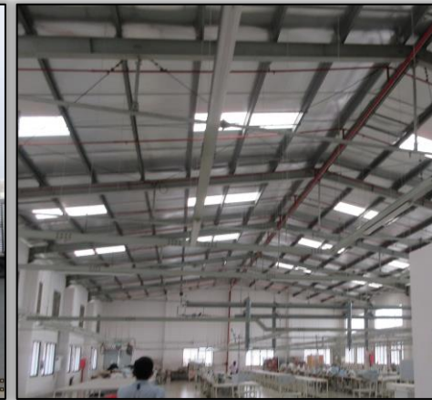
The sprinkler heads have been installed close to the ceiling under 400mm
