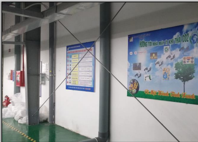
The column bracings have been installed
