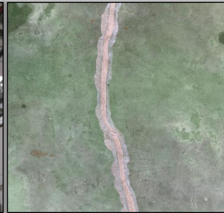
Cracks have been remediated by contractor
