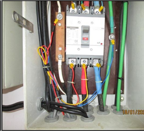
Small cables 2mm 2 connected to MCCB 250A
