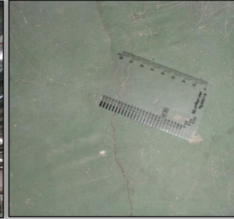
Cracks on the mezzanine floors
