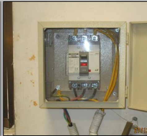
Suitable CB has been provided for small cables
