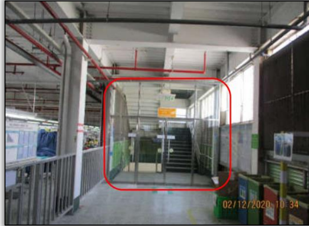
Inadequate fire rated enclosure of stairs for the multiple floors building
