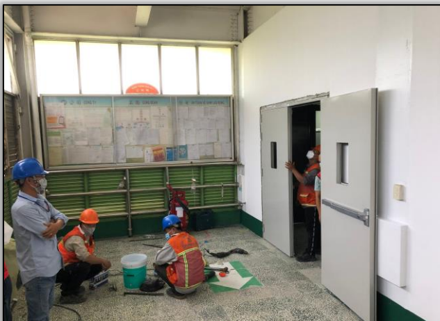
The fire rated protective enclosures to the stairs provided
