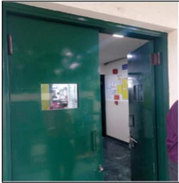
Wooden door installed on stair enclosure
