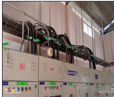
Cable identification has been given to all wiring.
