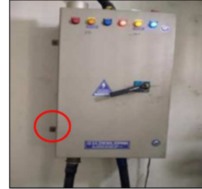
Body earthing not provided to electrical panel
