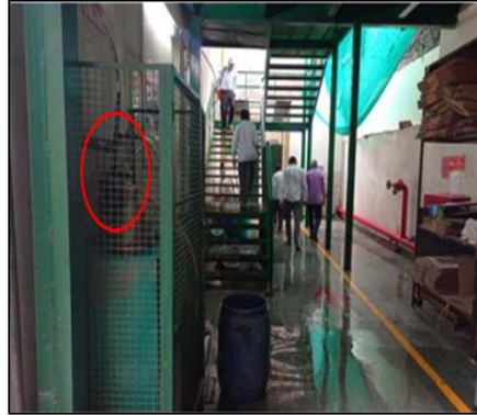
Diesel storage in evacuation path
