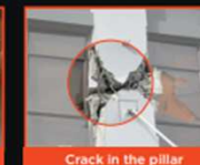
Crack in the pillar
