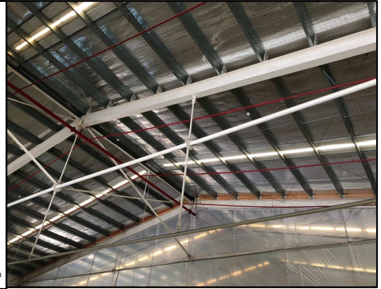
FIGURE 8.6.4.1.3.1(b) Sprinklers at Pitched Roof; Branch Lines Run Up Slopes.
