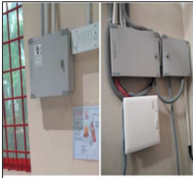
No identification of panels and cables
