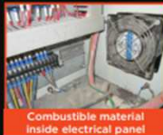
Lint/dirt on electrical panel
