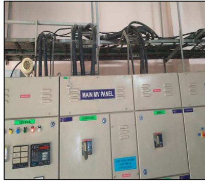
Electrical wiring and cables not properly identified
