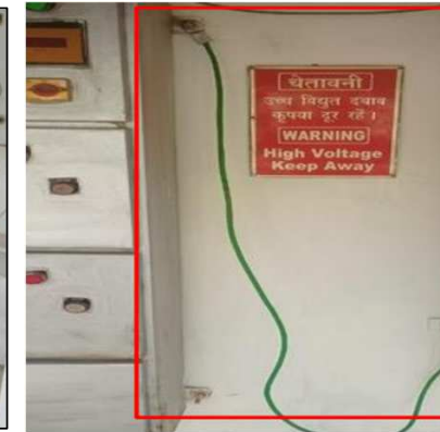
Body earthing provided to electrical panel
