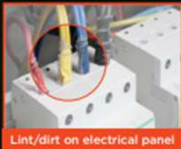
Lint/dirt on electrical panel
