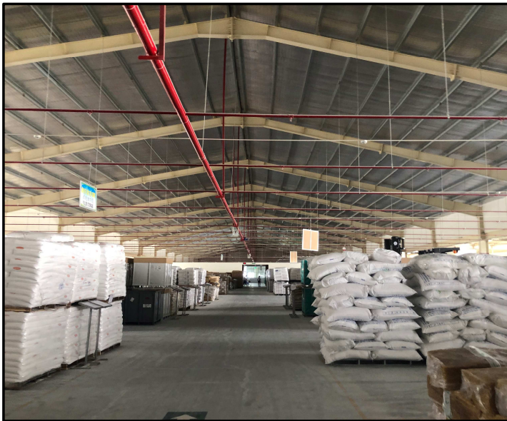
FIGURE 8.6.4.1.3.1(b) Sprinklers at Pitched Roof; Branch Lines Run Up Slopes.
