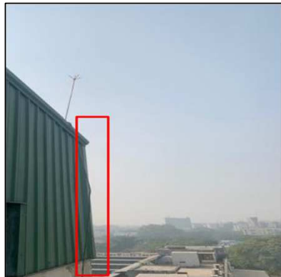
Earthing provided to MS truss
