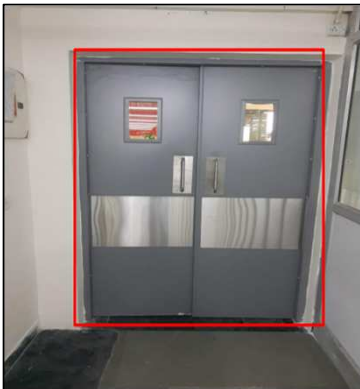
Fire rated doors installed
