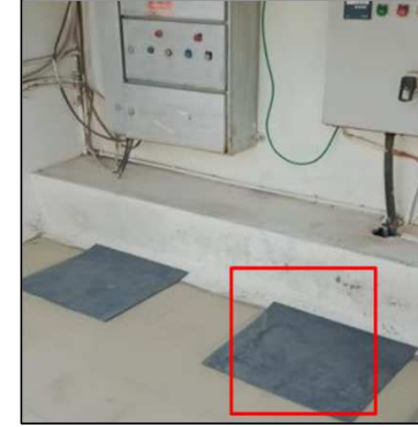
Electrical mats provided under electrical panel
