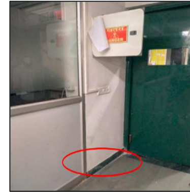
Insulated rubber mat not installed under electrical panel
