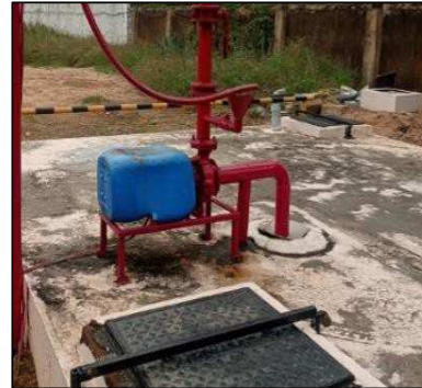
Single 7.5 HP pump installed for fire fighting
