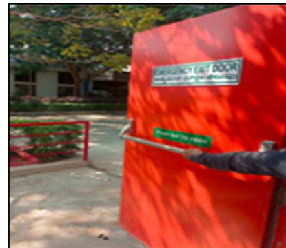
Rolling shutter replaced with fire rated doors with push bar
