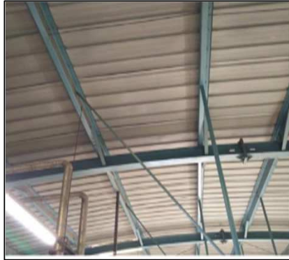
Earthing not provided to Ms truss
