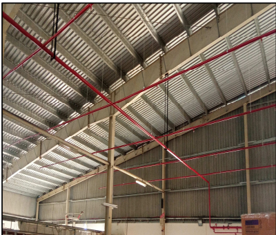
Sprinkler protection systems has been installed
