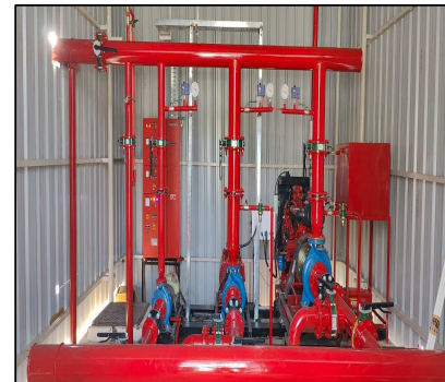
Jockey/Electrical/Diesel Operated pumps installed
