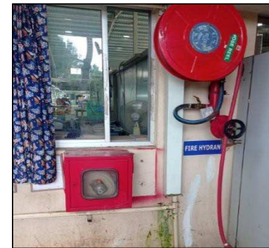
Hose pipe cabinet having single 15 meter length hose pipe
