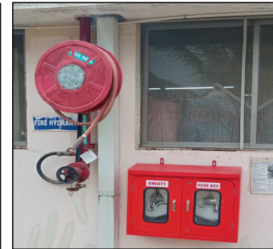
Double hose 2X15m Has been fixed all existing setup.
