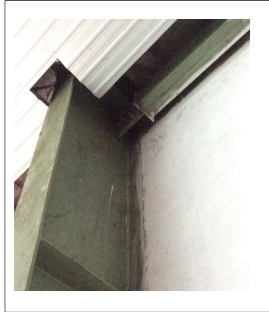
Figure N Typical eaves detail – eaves beam visible
