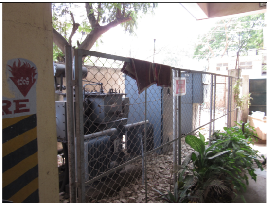
Figure 12 Diesel cooled Transformer adjacent Crèche and large window onto Stair
