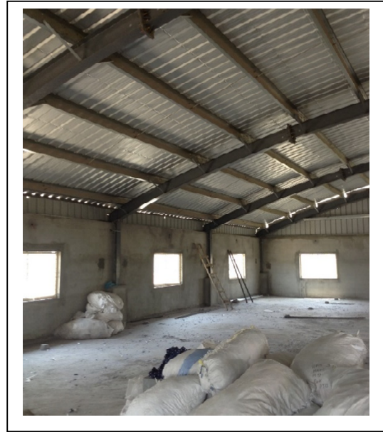
Figure 11 Additional steel structure on 4 th floor
