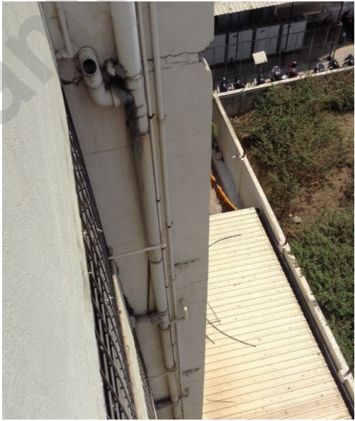
Figure 20 Cracks in cantilever at floor levels
