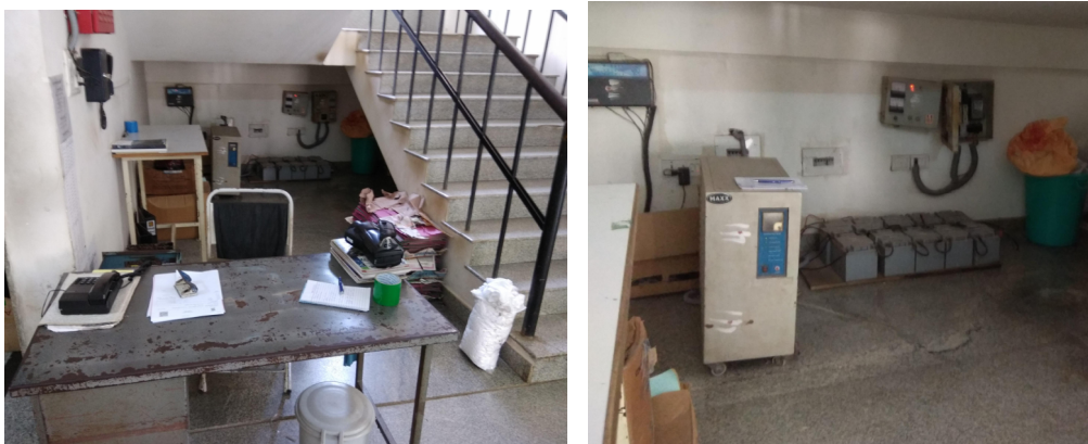
Figure 10 improper keeping of life safety UPS and its batteries.
