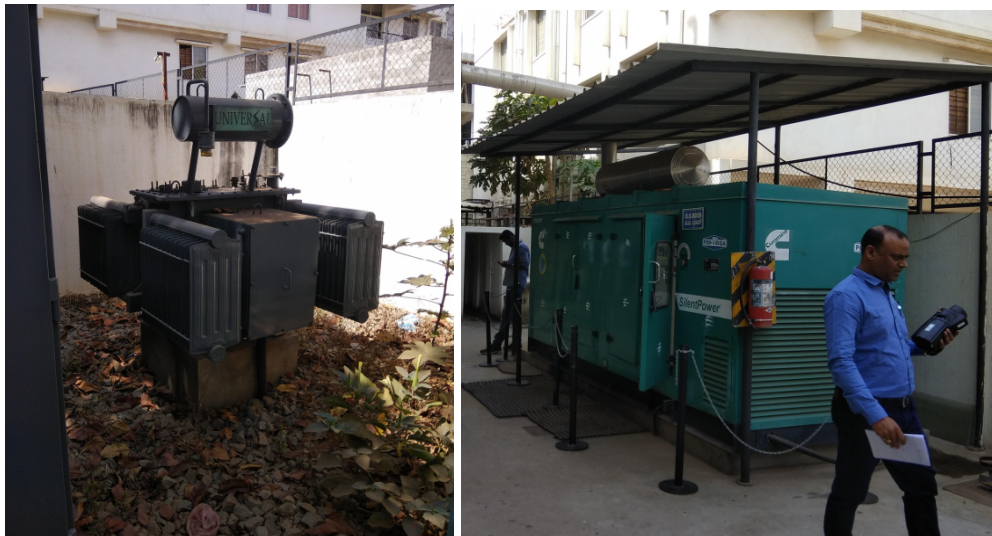
Figure N 250kVA Transformer and 200kVA DG set.
