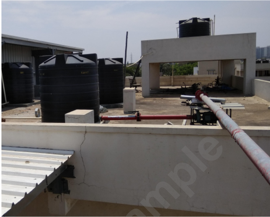
Figure 12 No proper human access to fire pump on terrace.
