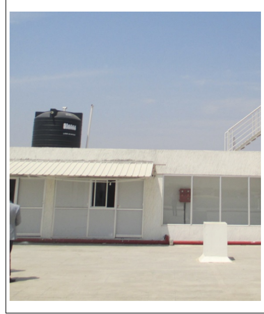
Figure N 10,000 litre tank at GL 0-11/D-E
