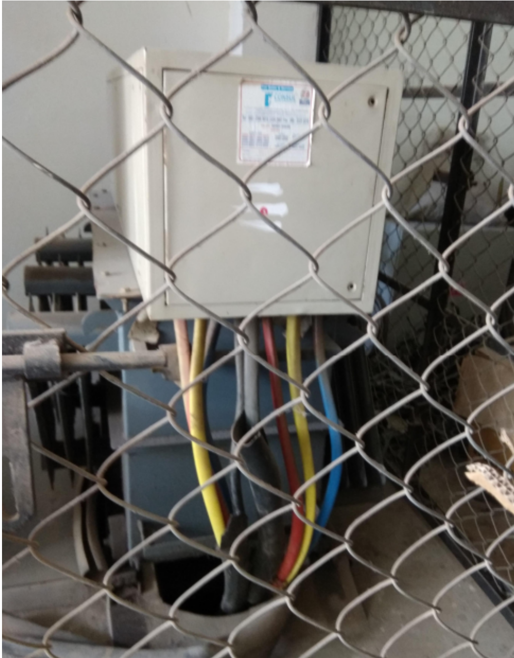
Figure N Improper termination of cables.
