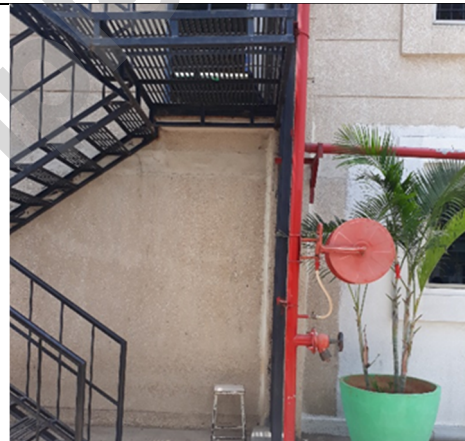
Figure 17 Hydrant connection and hosereel at discharge area SW Stair
