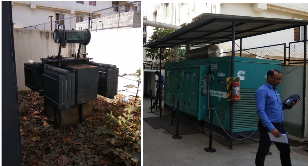
Figure 4 250kVA Transformer and 200kVA DG set.
