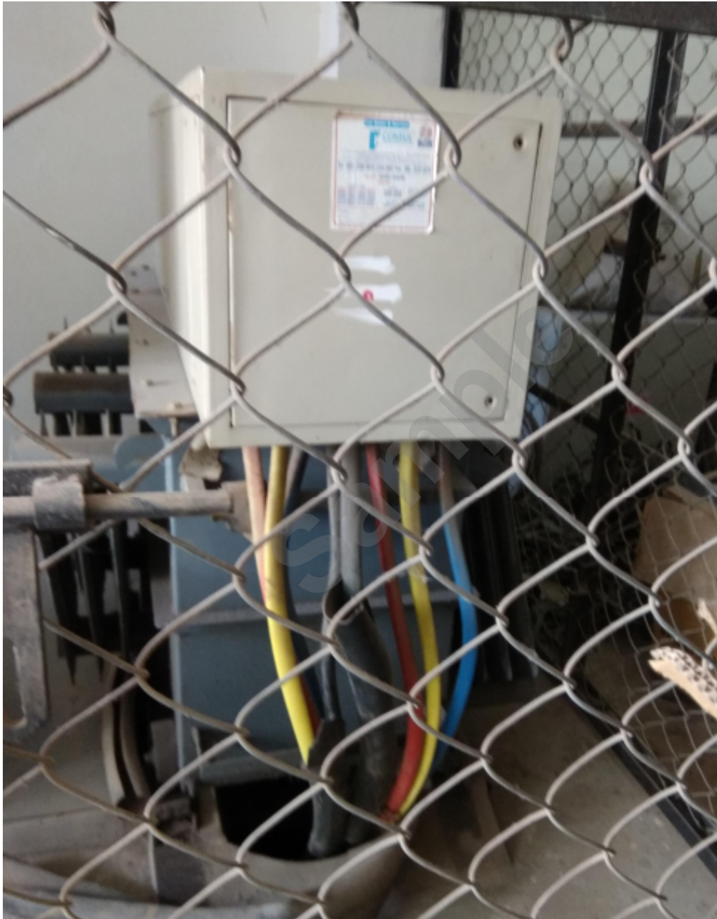
Figure 8 Improper termination of cables.
