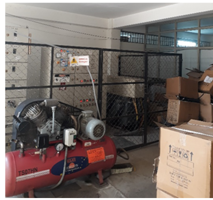
Figure 13 Carton box stored near HV Electrical Room
