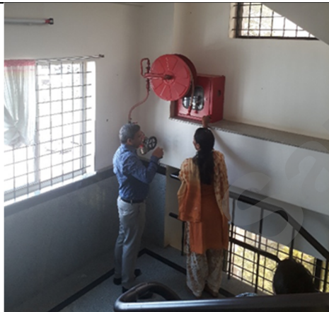
Figure 16 Fire hydrant and hose reel at half landing, located at height
