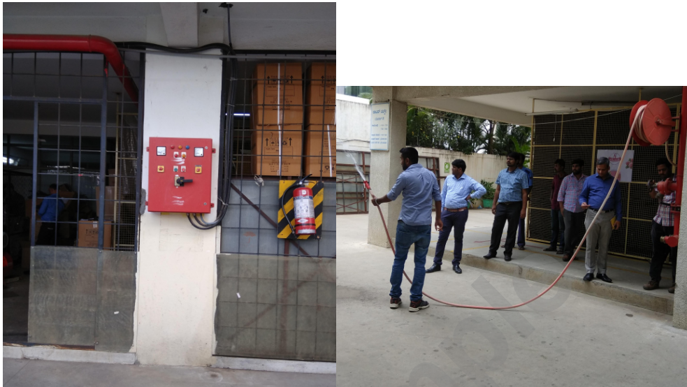
Figure 9 Manual operation of fire pump.
