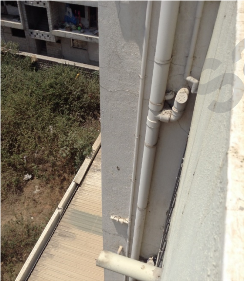
Figure 19 Cracks in cantilever area at floor levels
