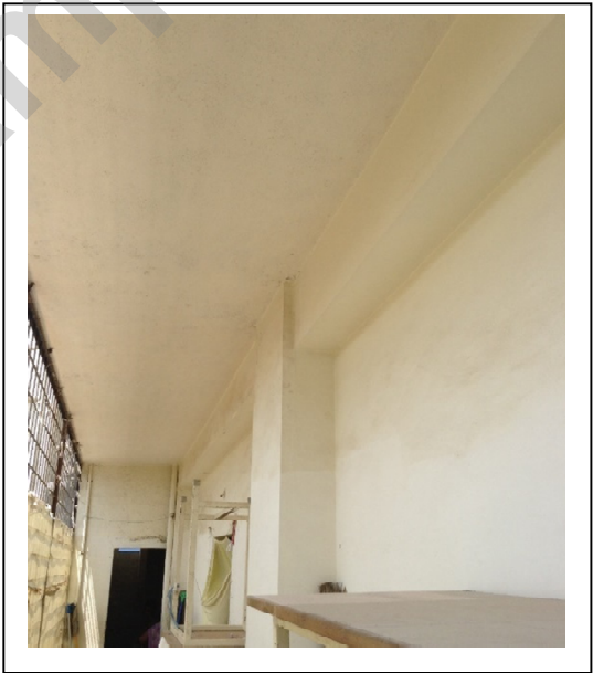
Figure 9 Typical slab cantilever to south elevation – 1.5m cantilever
