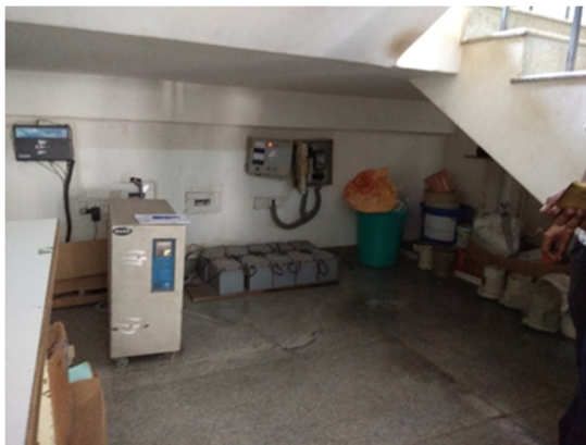
Figure 12 UPS and back-up batteries stored under NW Stair flight
