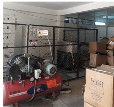
Figure 13 Carton box stored near HV Electrical Room
