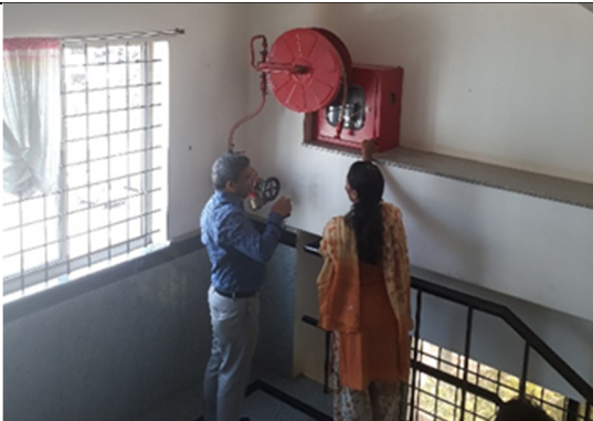
Figure 13 Fire Hydrant and hose reel at half landing, located at height (eg. above)
