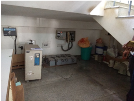
Figure 10 Miscellaneous storage and UPS battery back-up under stairway (eg. above)
