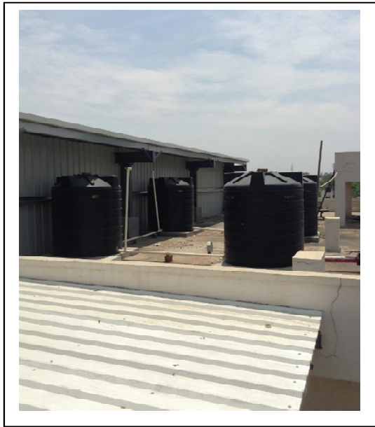
Figure 10 Water tanks on terrace – 4 no. 3000l tanks and 2 no. 2000l tanks
