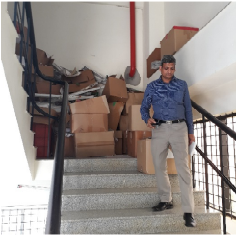
Figure 10 Evacuation pathways obstructed by uncontrolled storage
