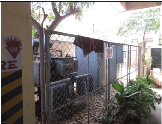
Figure 12 Diesel cooled Transformer adjacent Crèche and large window onto Stair (eg. above)
