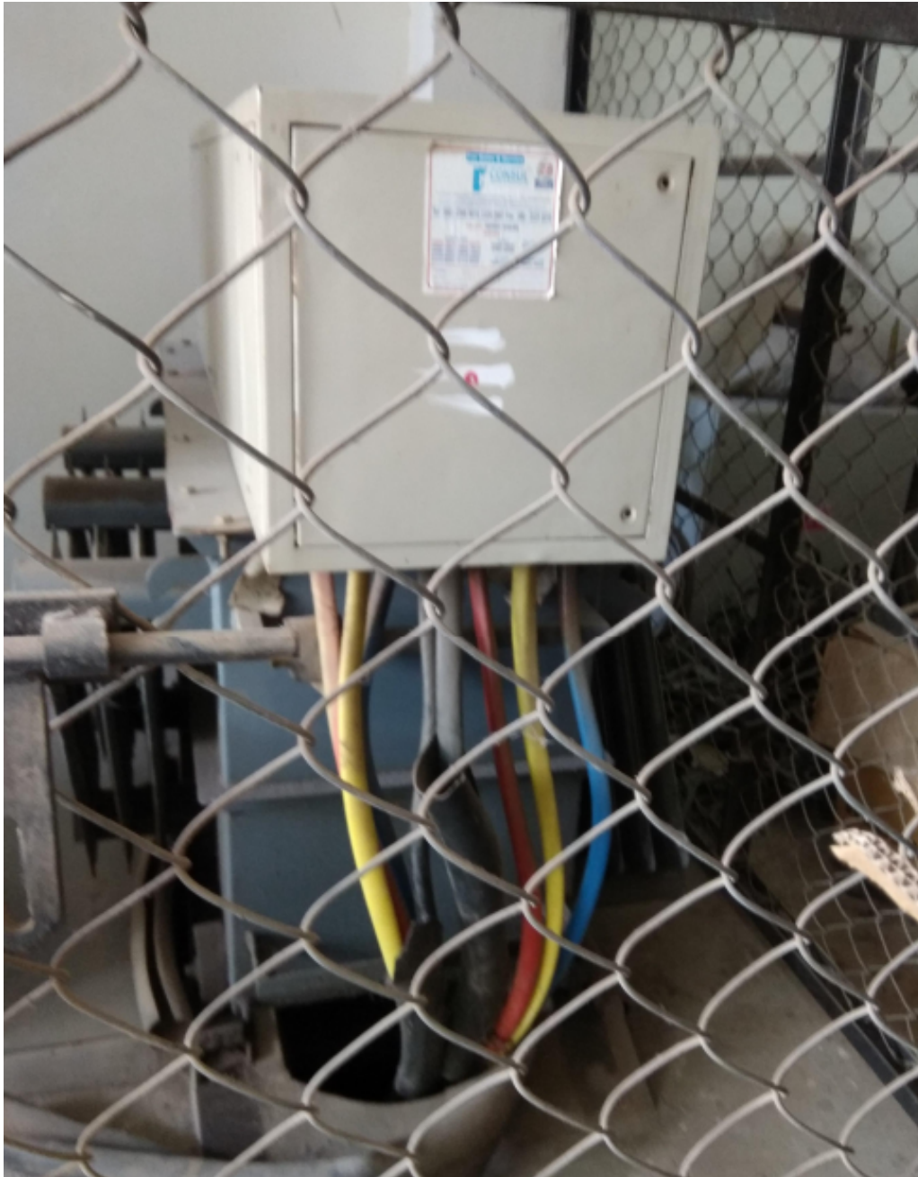
Figure N Improper termination of cables.
