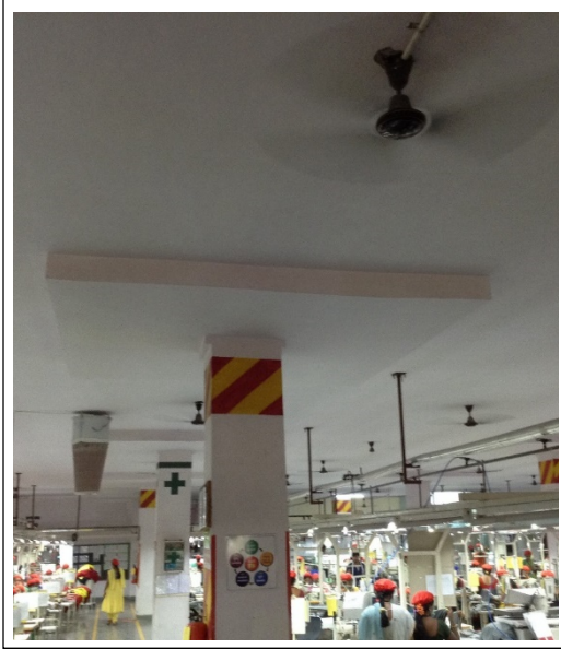
Figure N Typical flat slab with drop panels
