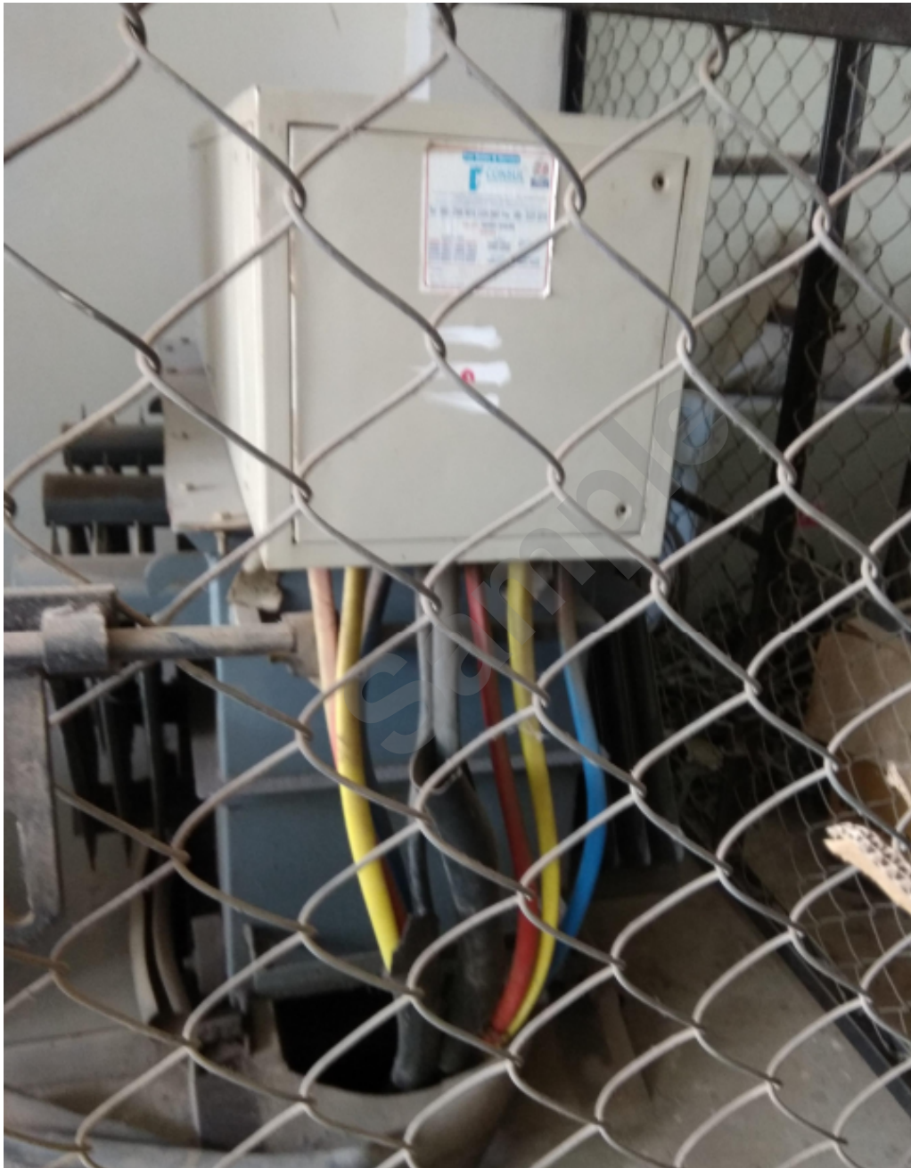
Figure 8 Improper termination of cables.
