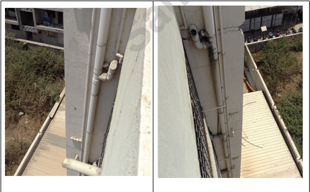
Figure 19 Cracks in cantilever area at floor levels
