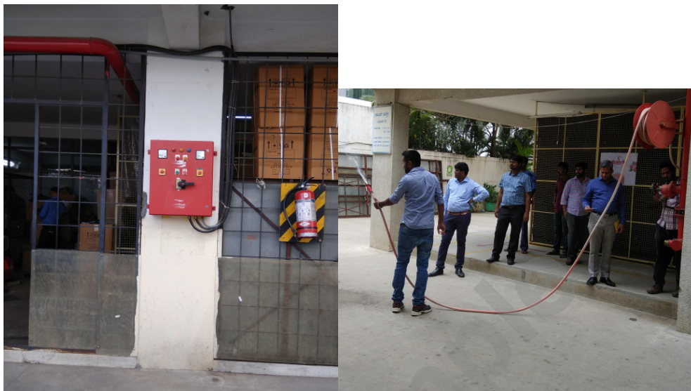
Figure 9 Manual operation of fire pump.
