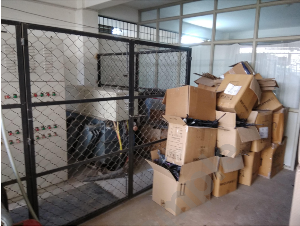
Figure 6 Storage of combustible material near main LY panel metal fencing.
