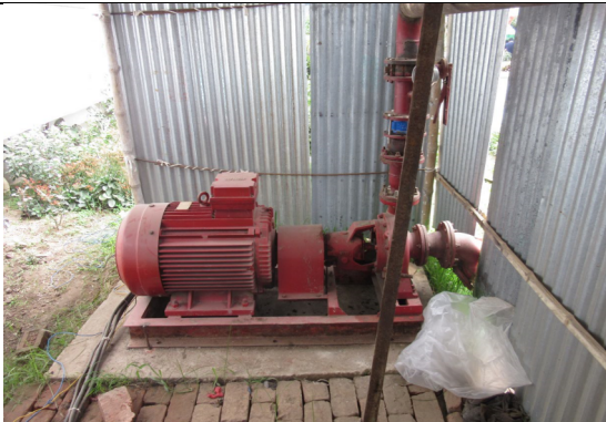
Figure 14 Centrifugal suction fire water pump adjacent to reservoir (eg. above)
