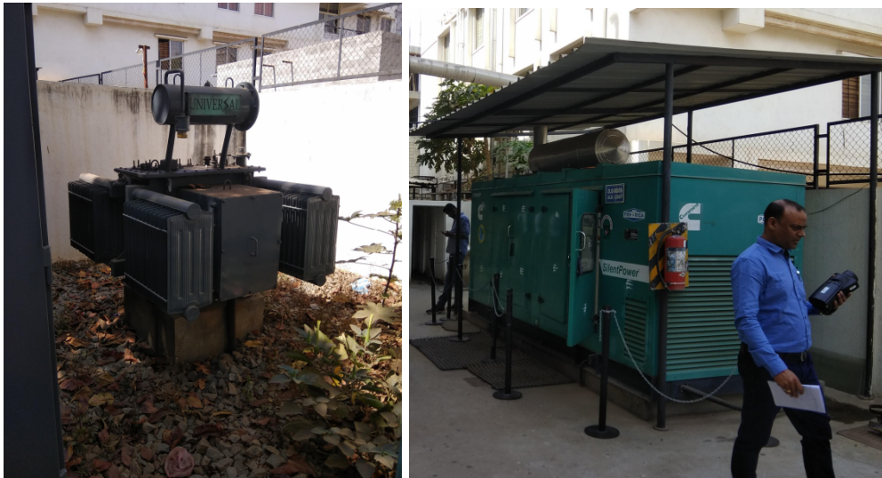
Figure 4 250kVA Transformer and 200kVA DG set.
