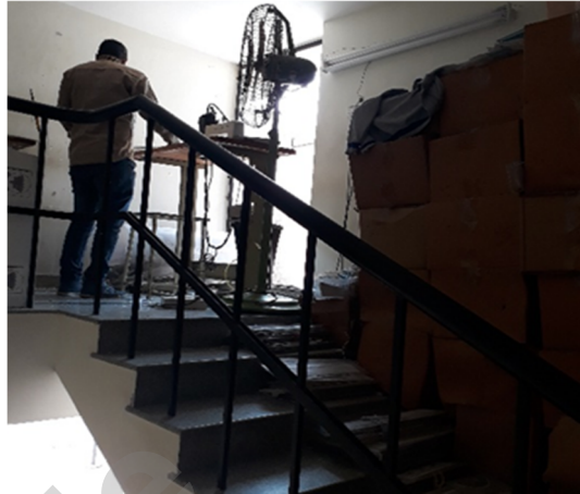
Figure 11 Evacuation pathways obstructed by uncontrolled storage
