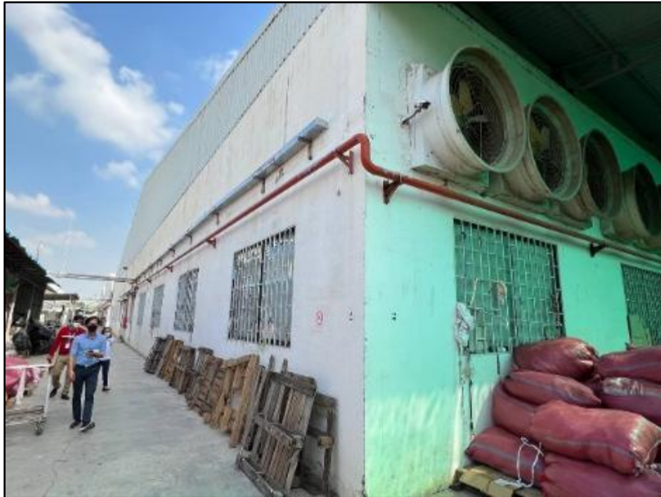
Figure 5: West Side View
