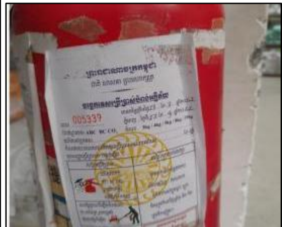
Figure11: Fire Extinguisher was not checked regularly at Dormitory
