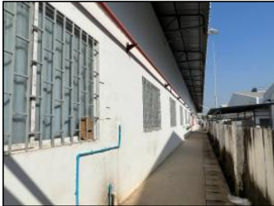
Figure 7: Building C – East Side View
