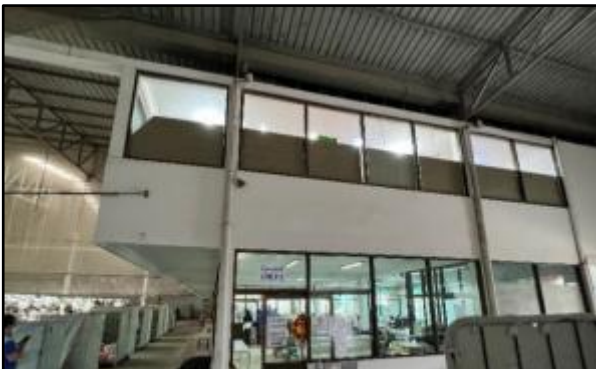
Figure 24: Cantilever floor of building A
