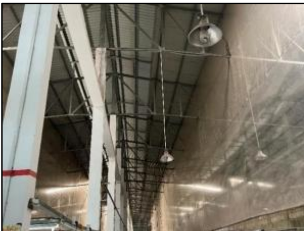
Figure 23: Truss system supported by concrete columns
