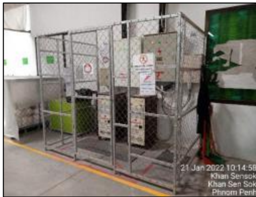
Figure 23: Distribution Boards (DBs) insides building A.
