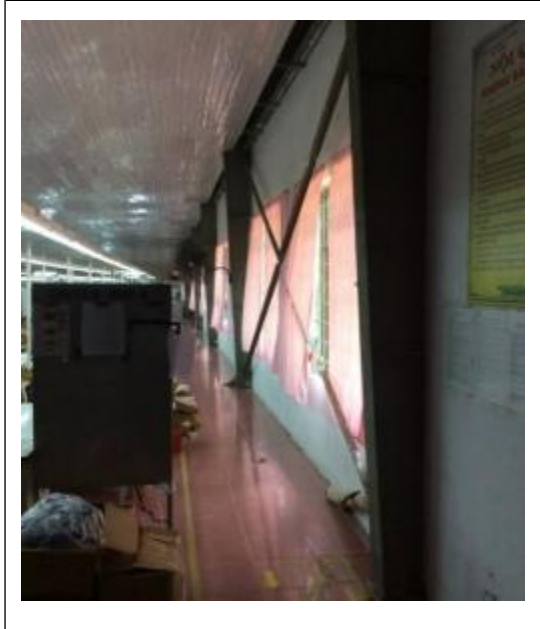
Figure N Typical braced bay – suspended ceilings throughout so portal frames not visible. External masonry wall built tight to outside of column flange
