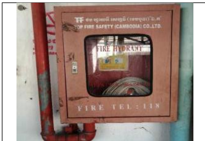
Figure 13 Fire Hydrant and hose reel at half landing, located at height
