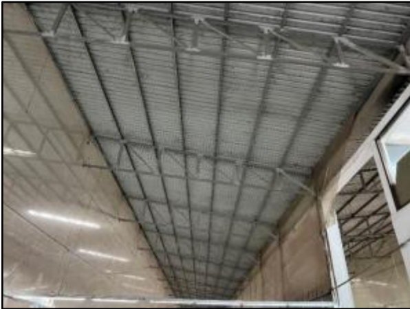
Figure 22: Roof truss system of building A
