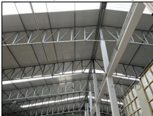
Figure 30: Zoom-in view of the truss system supported by the columns
