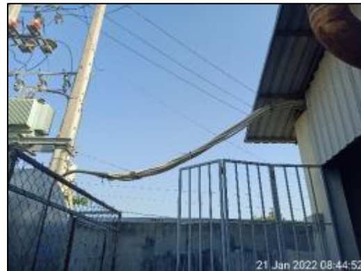
Figure 17: Pole mounted oil type transformers at outside of Factory Boundary (Belong to EDC) with overhead LV cables to LVMSB/MTS panel in Generator Room 01 near Building A.
