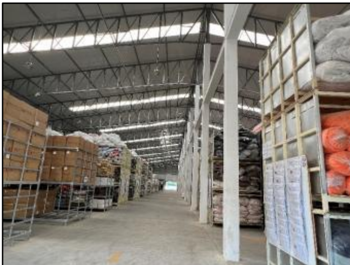
Figure 29: Truss system of the building
