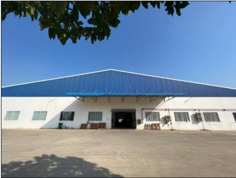
Figure 5: Front view of Building C
