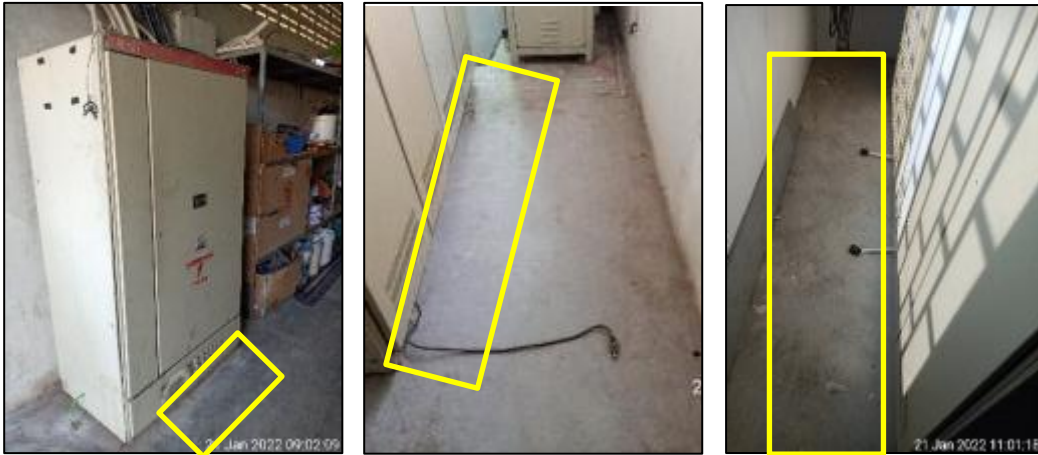
Figure 46: Inadequate rubber floor mats for MTS-01 panel, MDBS & DBs panel.
