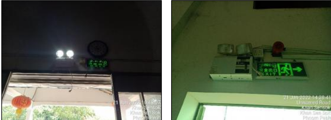
Figure 8: Emergency & Exit Lighting Testing Time at Building A
