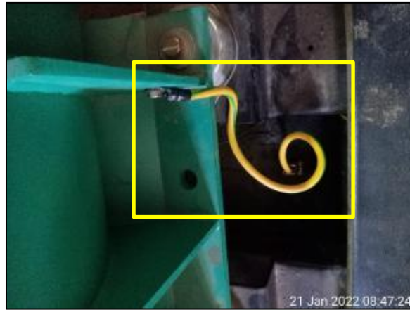
Figure 11: Incorrect size PE Earthing cable for generator at generator room.
