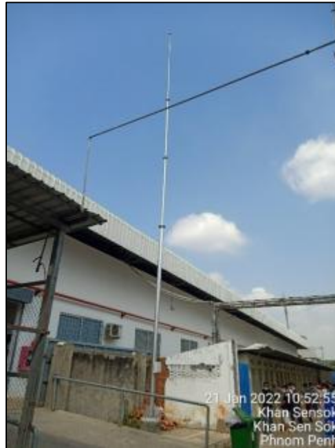
Figure 16: Lightning Protection System Air Terminal Zone 02 installed on Steel Pole near Building C with earthing resistance testing report.
