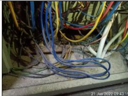
Figure 60: Lint and Dust in MDB-001B.
