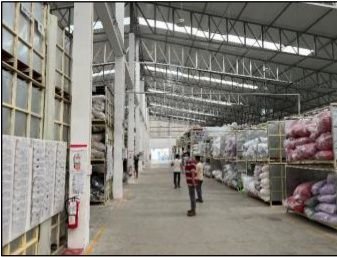
Figure 28: Inside view of the structural system
