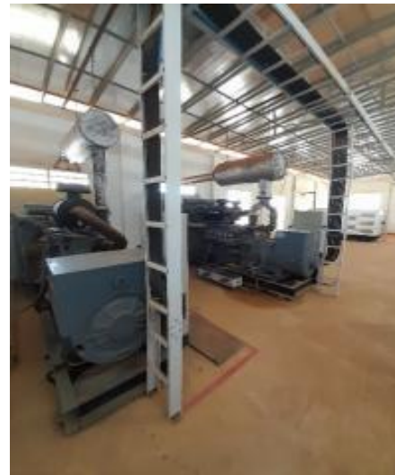
Figure N 250kVA Transformer and 200kVA DG set.
