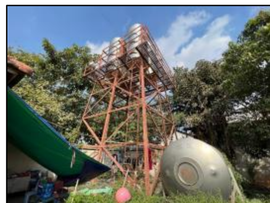
Figure 10: Water Tanks – Side View
