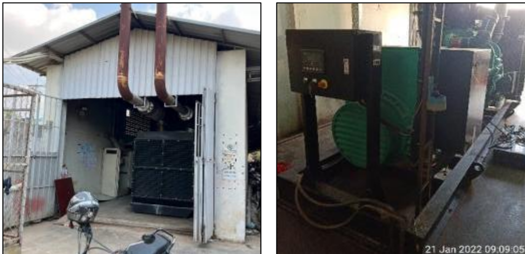
Figure 19: 900kVA Generator Room 01 without ventilation fan near Building A.
