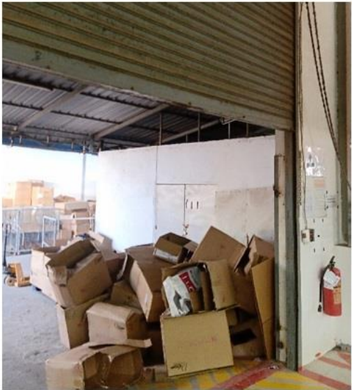
Figure 8 Temporary storage of carton along the Exits (e.g. Above)
