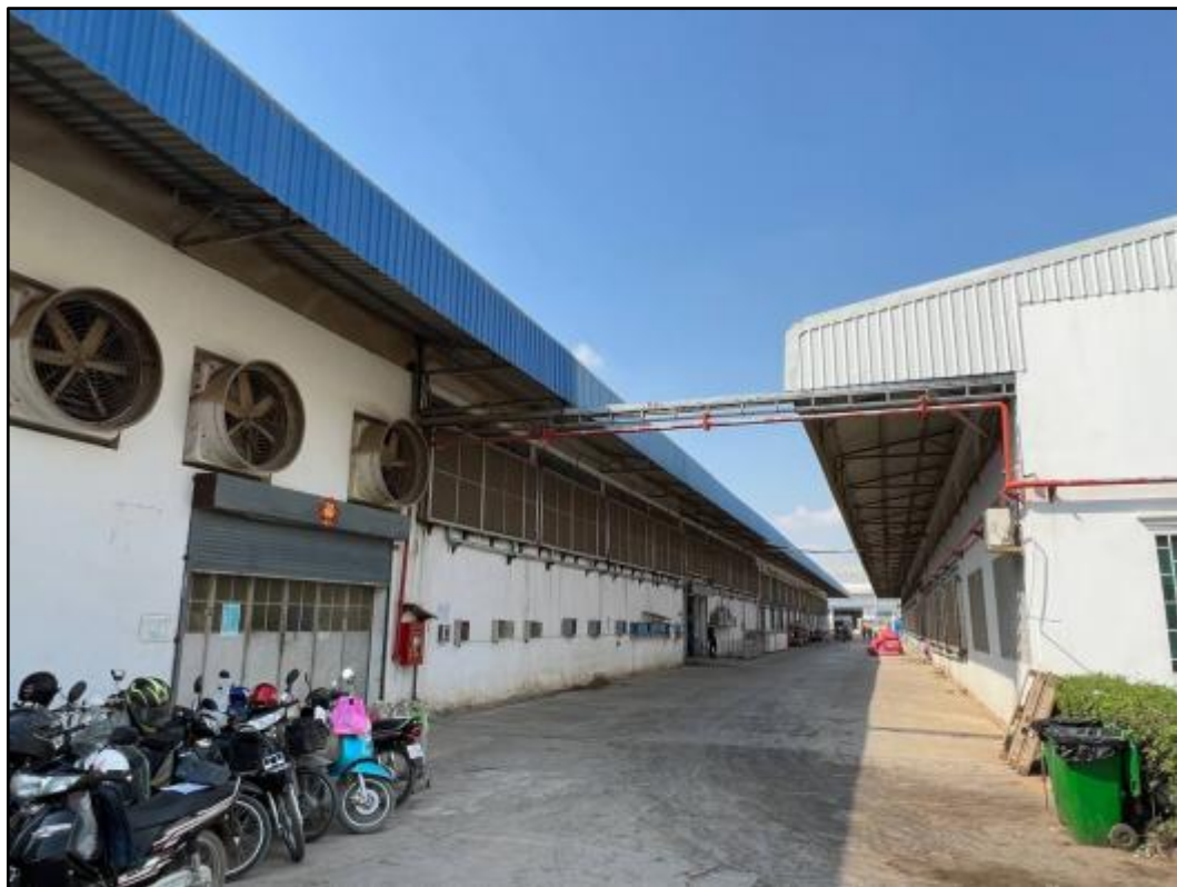
Figure 4: Building B – Front view
