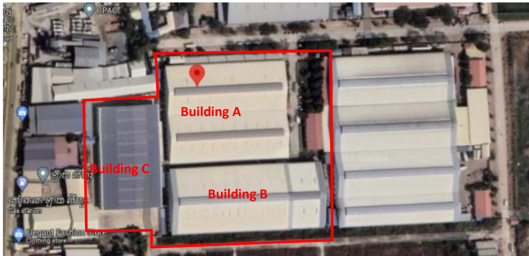
Figure 1: Satellite Image of the Factory
