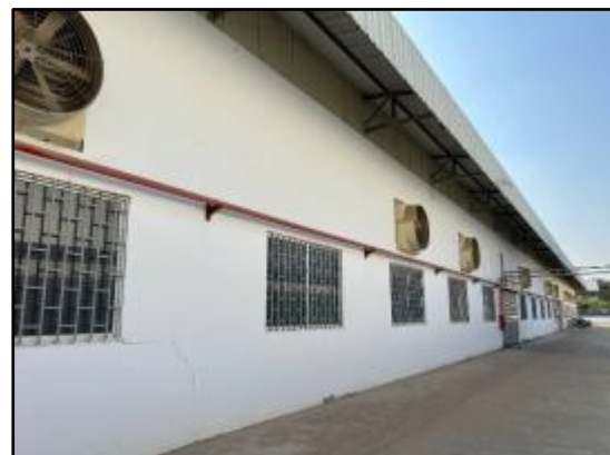
Figure 8: Building C – West Side View
