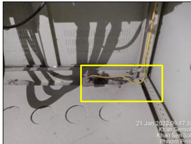
Figure 14: Missing PE Earthing bar installation for Electrical panel at building A
