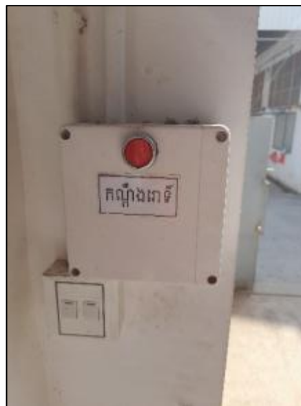
Figure 10: Fire Detection & Alarm (MCPs) tested at Building C.
