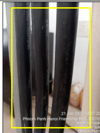
Figure 54: Under size of phases cable cross-sectional area compare to circuit breaker from Generator 02 panel to ATS panel inside Building C.
