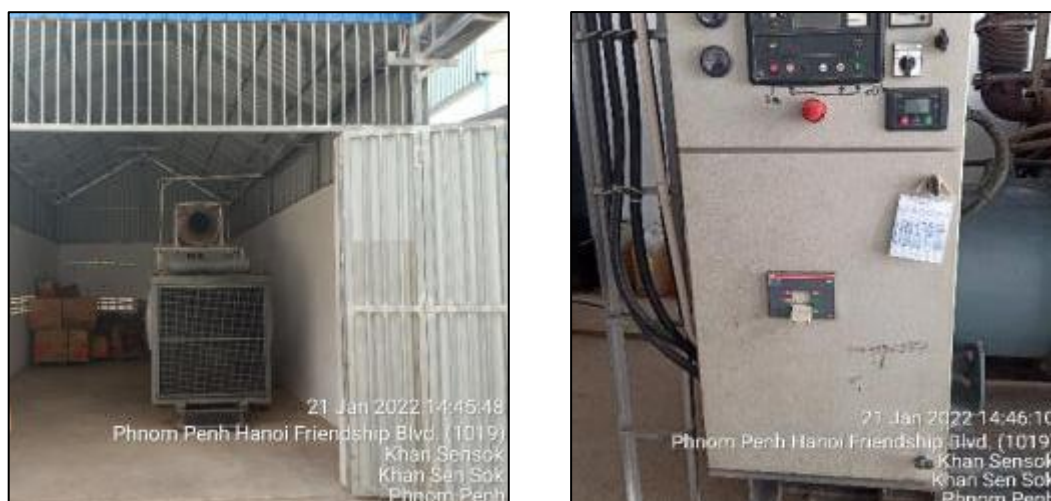
Figure 21: 500kVA Generator Room 02 without fan ventilation system at behind Building C.
