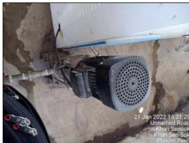
Figure 35: No Earthing bonding cable connected to boiler and pump boiler enclosure.
