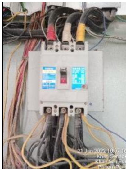
Figure 61: Lint and Dust in DB-004B
