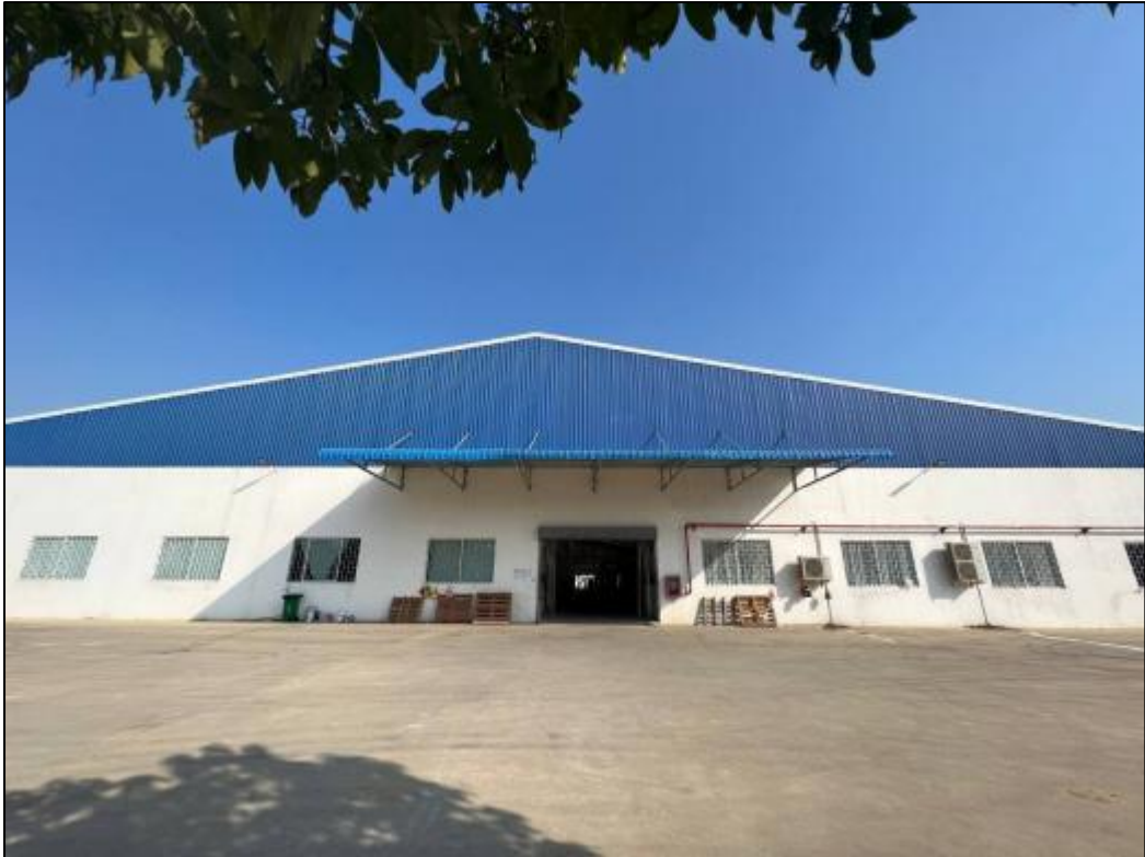
Figure 5: Front view of Building C
