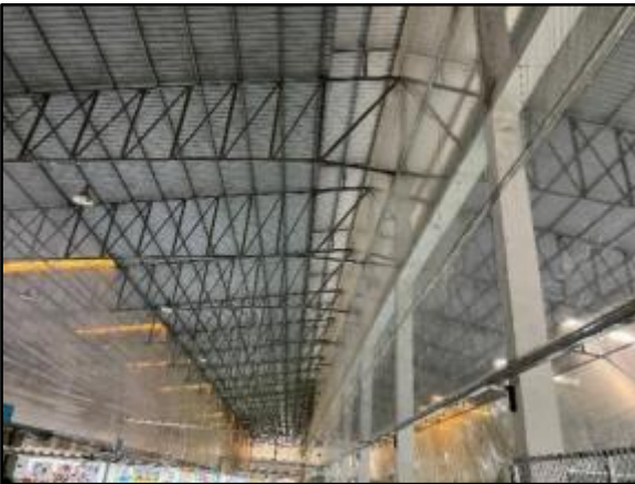
Figure 26: Roof truss system of building B
