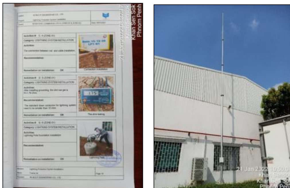
Figure 15: Lightning Protection System Air Terminal Zone 01 installed on Steel Pole near Building A with earthing resistance testing report.
