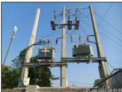
Figure 17: Pole mounted oil type transformers at outside of Factory Boundary (Belong to EDC) with overhead LV cables to LVMSB/MTS panel in Generator Room 01 near Building A.
