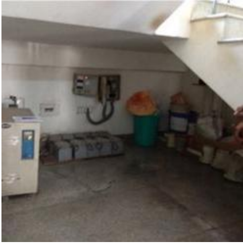
Figure 10 Miscellaneous storage and UPS battery back-up under stairway
