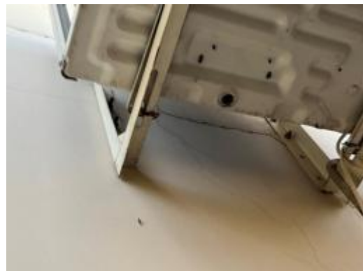
Figure 45: Wall cracking at Hostel building
