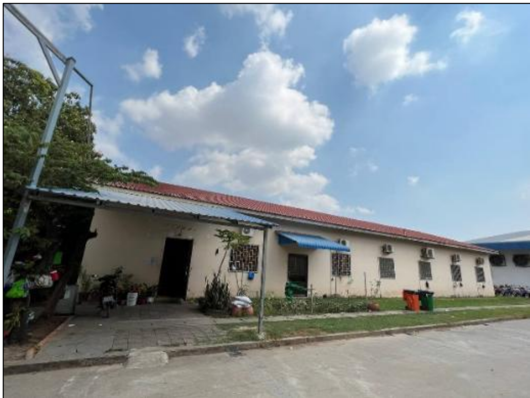
Figure 6: Hostel Building overview
