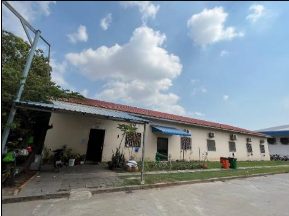
Figure 6: Hostel Building overview
