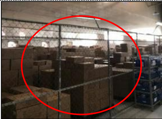
Figure 28: Separation of different occupancies was incomplete between finished goods storage at building B
