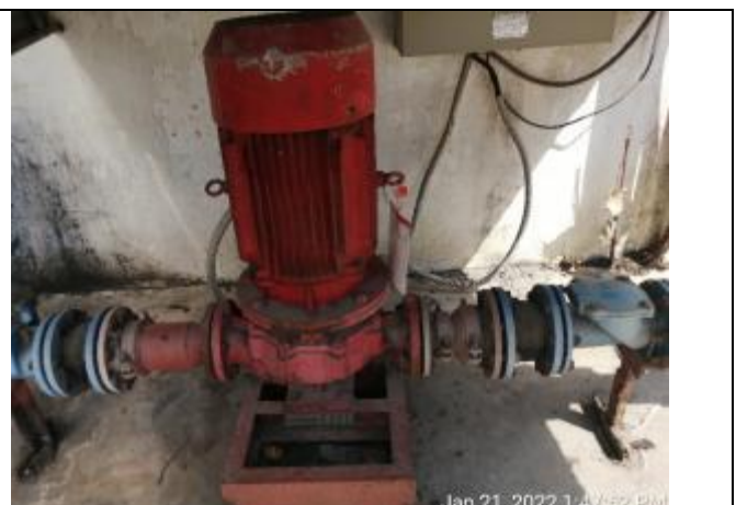
Figure 14 Centrifugal suction fire water pump adjacent to reservoir
