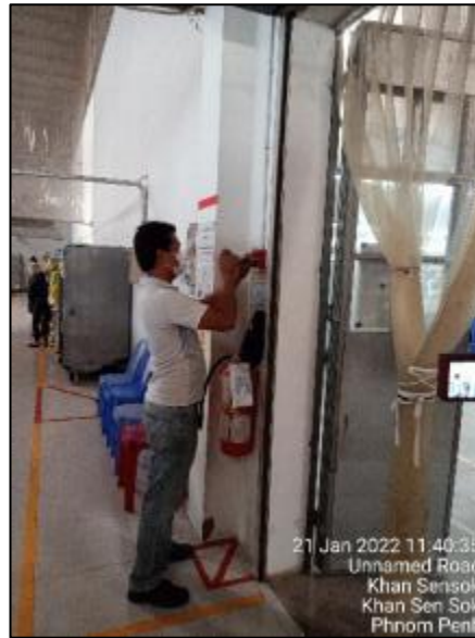
Figure 9: Fire Detection & Alarm (MCPs) tested at Building B.
