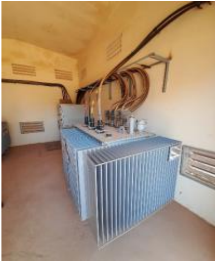
Figure N 250kVA Transformer and 200kVA DG set.
