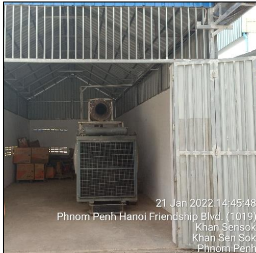
Figure 21: 500kVA Generator Room 02 without fan ventilation system at behind Building C.
