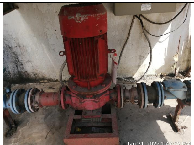
Figure 14 Centrifugal suction fire water pump adjacent to reservoir
