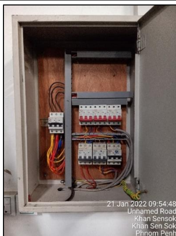
Figure 47: Combustible/flammable materials (wood) installed in SDB-001B.
