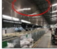
F3.1.2.1_Inadequate smoke detector.JPG
