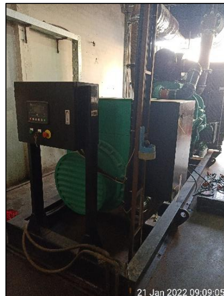
Figure 40: Insufficient generator 01 earthing with two separate points.
