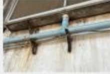
STR10 Steel support corrosion at building B.JPG
