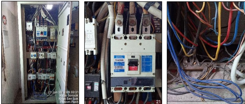
Figure 49: Inadequate cable segregation for LV cables inside MDB-001B
