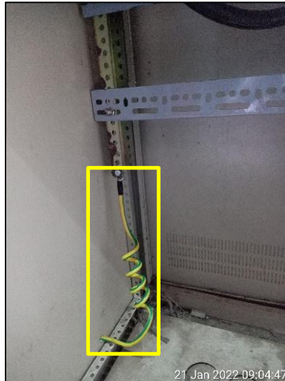
Figure 13: Incorrect PE Earthing cable installation for Electrical panel at building A
