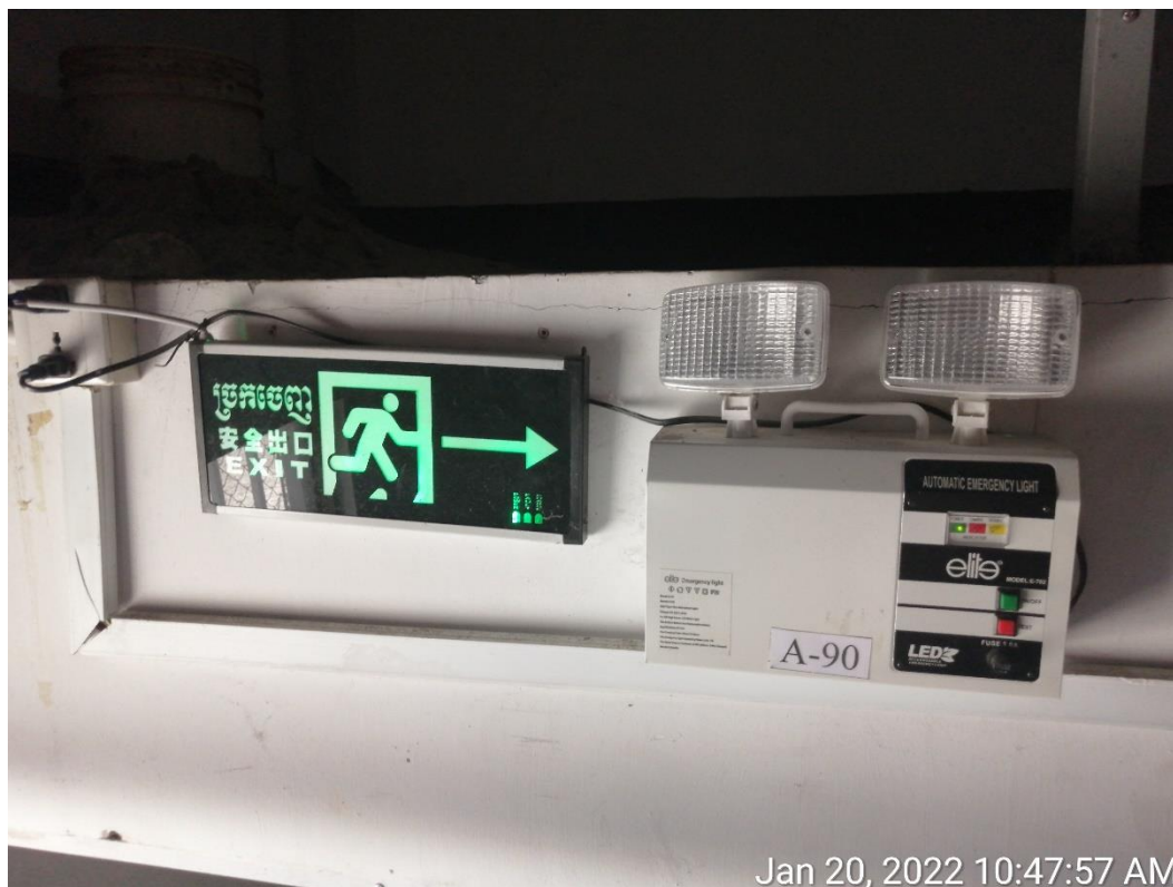
Figure N Emergency Lighting
