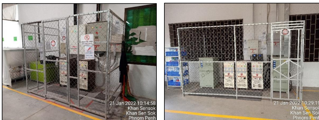
Figure 23: Distribution Boards (DBs) insides building A.
