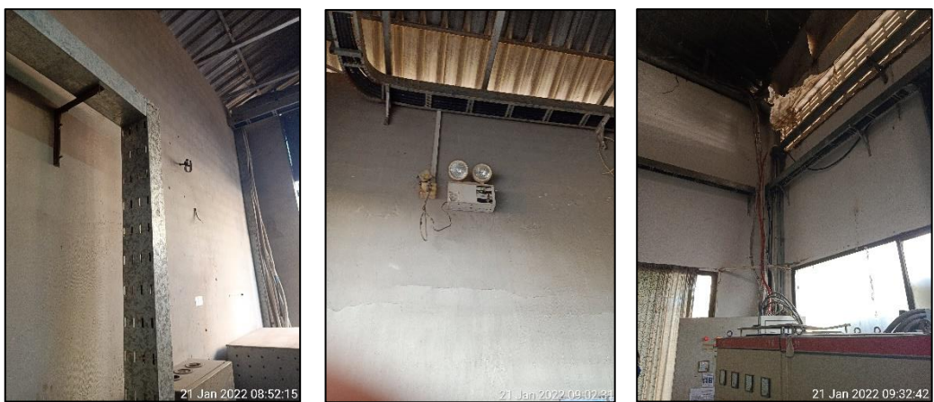
Figure 31: No Earthing bonding cable connected to cable routing (Tray, Ladder, Trunking...)
