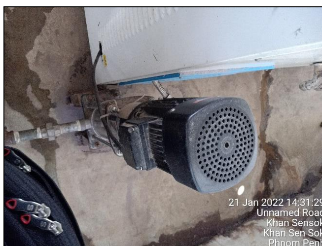
Figure 35: No Earthing bonding cable connected to boiler and pump boiler enclosure.
