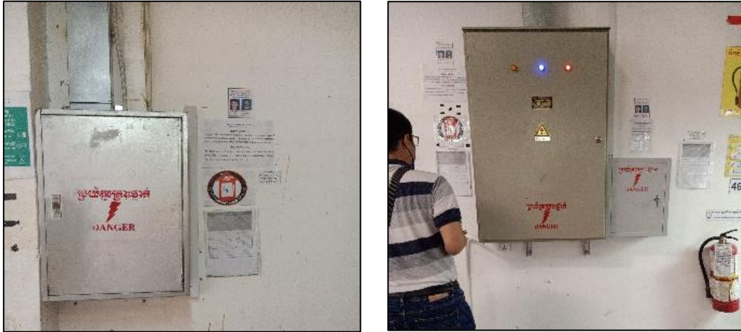
Figure 26: Sub-Distribution Boards (SDBs) inside Building B.
