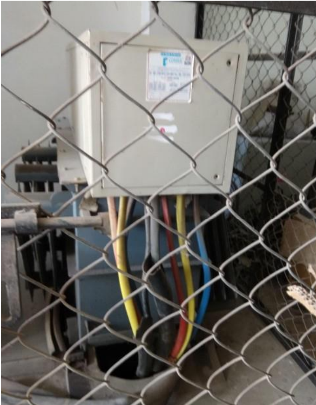
Figure N Improper termination of cables.
