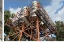
STR10 Corrosion on steel structure at water tank.jpg
