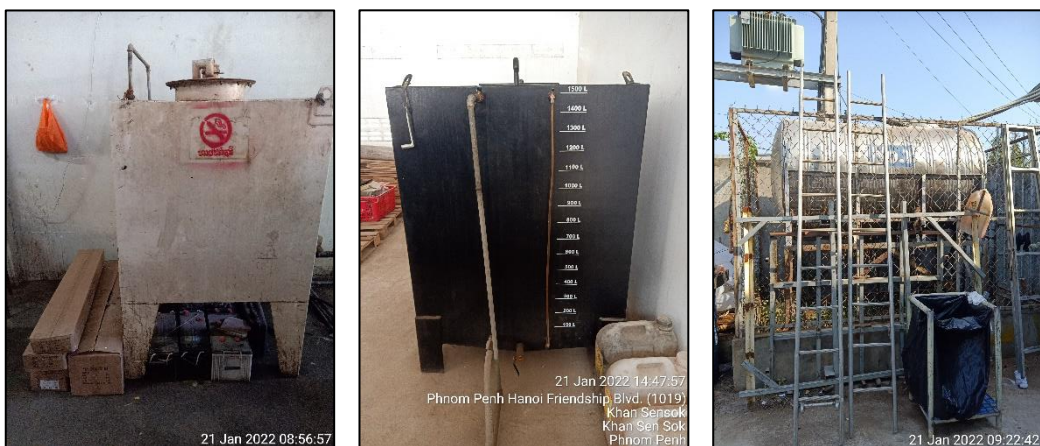
Figure 32: No Earthing bonding cable connected Fuel Daily Tanks and Bulk fuel storage tank.
