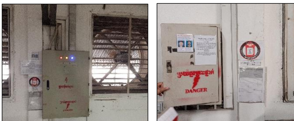
Figure 24: Sub Distribution Boards (SDBs) inside building A.
