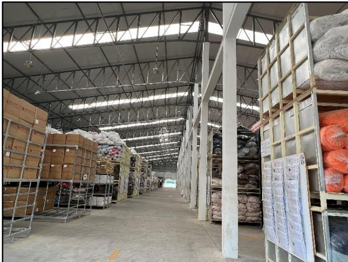
Figure 29: Truss system of the building
