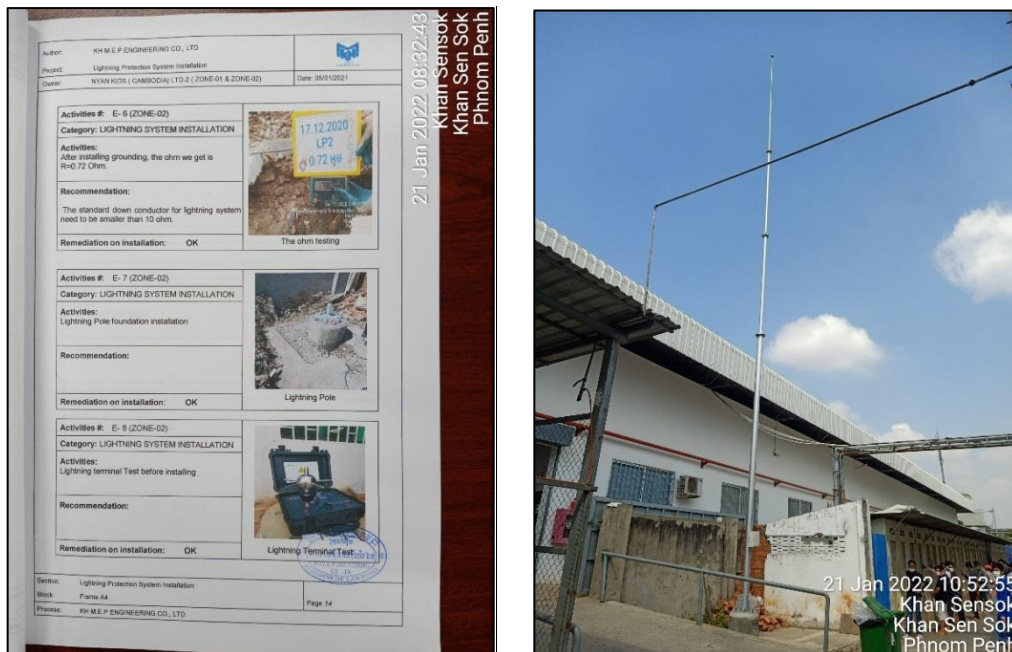
Figure 16: Lightning Protection System Air Terminal Zone 02 installed on Steel Pole near Building C with earthing resistance testing report.
