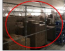
F2.2.2.1_Storage was incomplete separation.JPG
