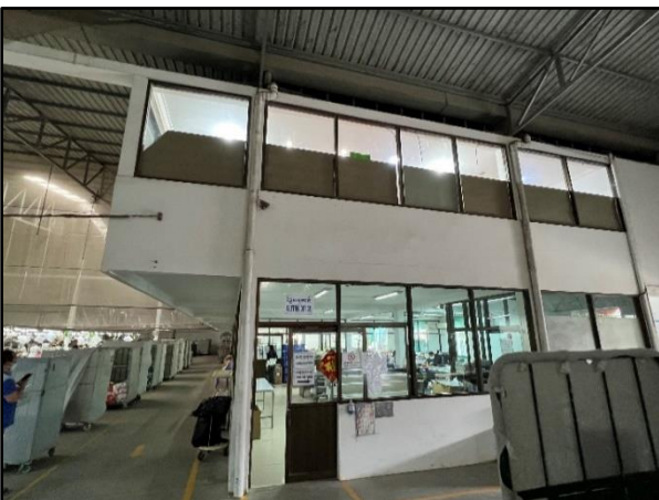
Figure 24: Cantilever floor of building A
