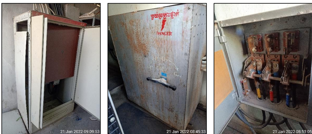
Figure 33: No Earthing bonding cable connected Electrical Panel Door Frames in Generator Room 01.
