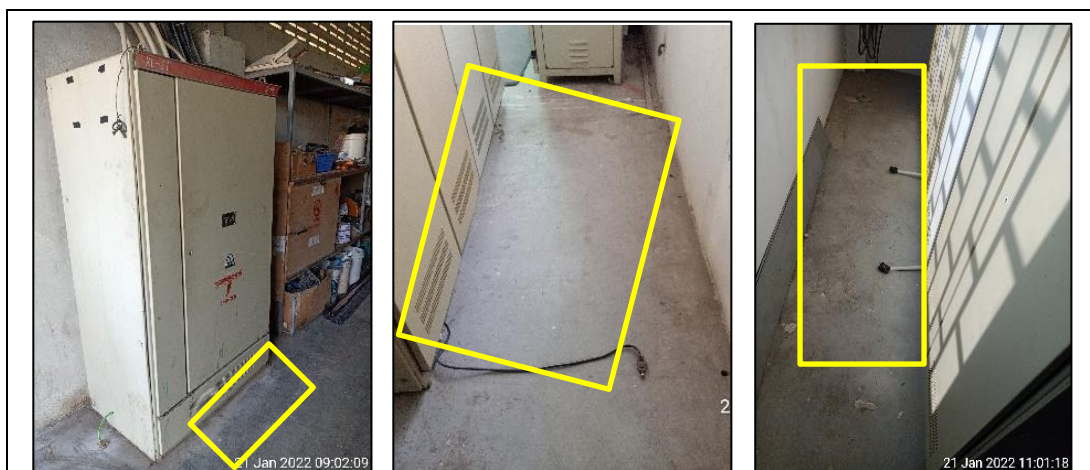
Figure 46: Inadequate rubber floor mats for MTS-01 panel, MDBS & DBs panel.
