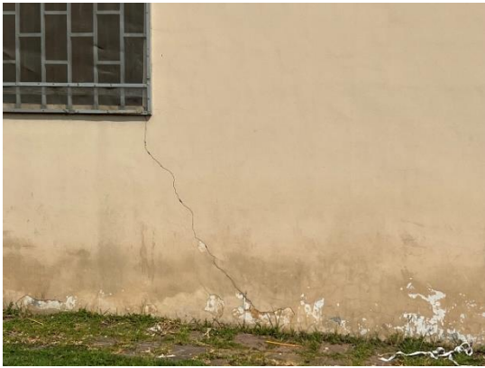
Figure 45: Wall cracking at Hostel building
