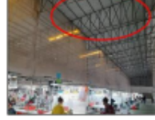
F3.1.2.2_Inadequate smoke detector.JPG
