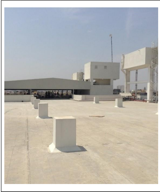
Figure N Water tank on columns at Roof level – GL E/7-8. Approx. storage – 24,000 liters Similar tank at GL E/2-3
