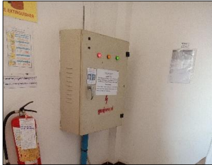
Figure 28: Distribution Board (DB) inside Hostel Building.
