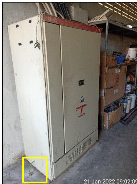
Figure 12: Incorrect size PE Earthing cable for generator panel at generator room.
