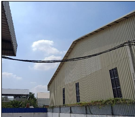
Figure 18: Incoming Overhead LV cables from another 400kVA Pole mounted oil type transformer to LVMSB/ATS panel in Electrical Room inside Building C.
