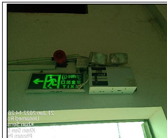
Figure 10: Inadequate back up power to emergency lighting
