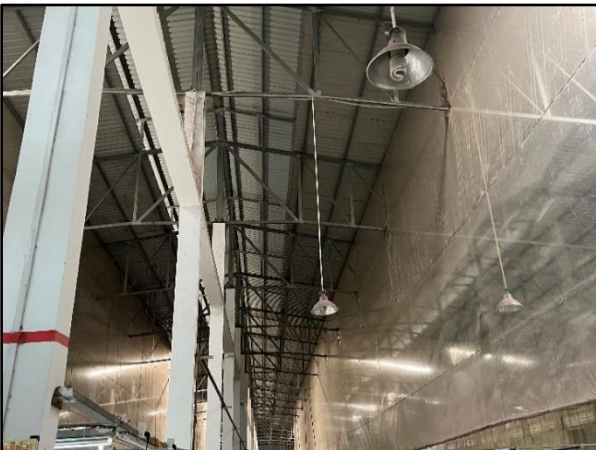
Figure 23: Truss system supported by concrete columns
