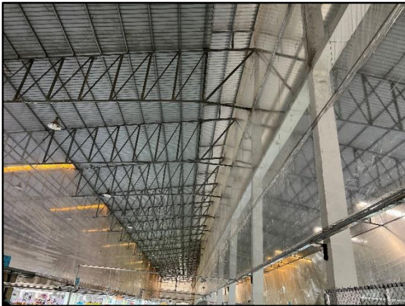
Figure 26: Roof truss system of building B
