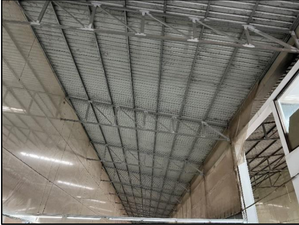
Figure 22: Roof truss system of building A
