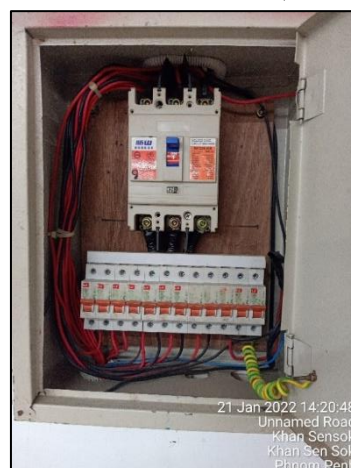
Figure 47: Combustible/flammable materials (wood) installed in SDB-001B.
