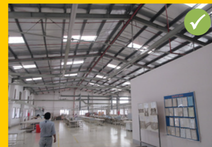
Sprinkler system re-installed closer to ceiling
