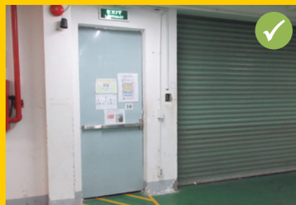
Locking mechanism replaced with push bar door mechanism
