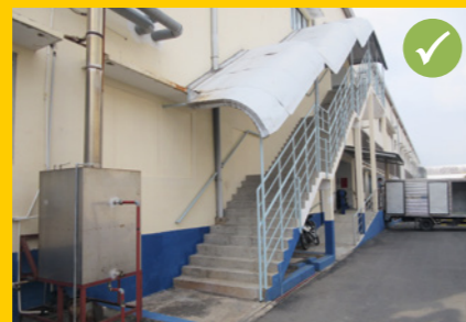
Fire rated enclosure provided for staircase
