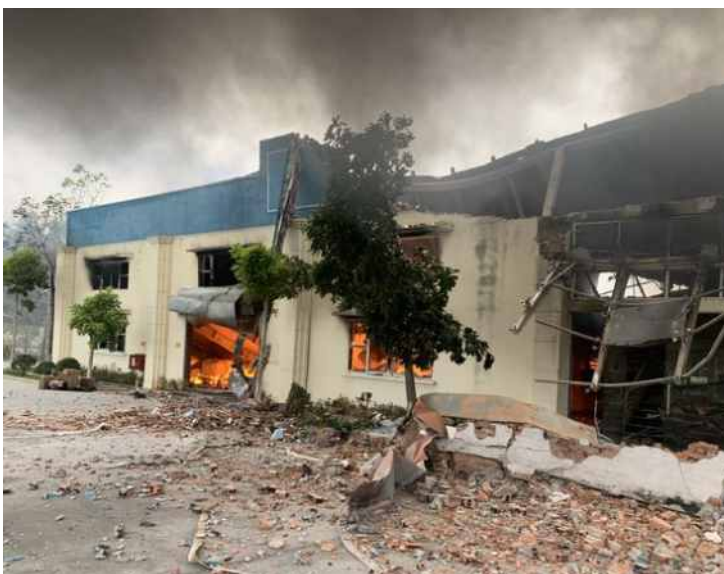
Fire Incident at Ivory Trieu Son factory, North Vietnam
